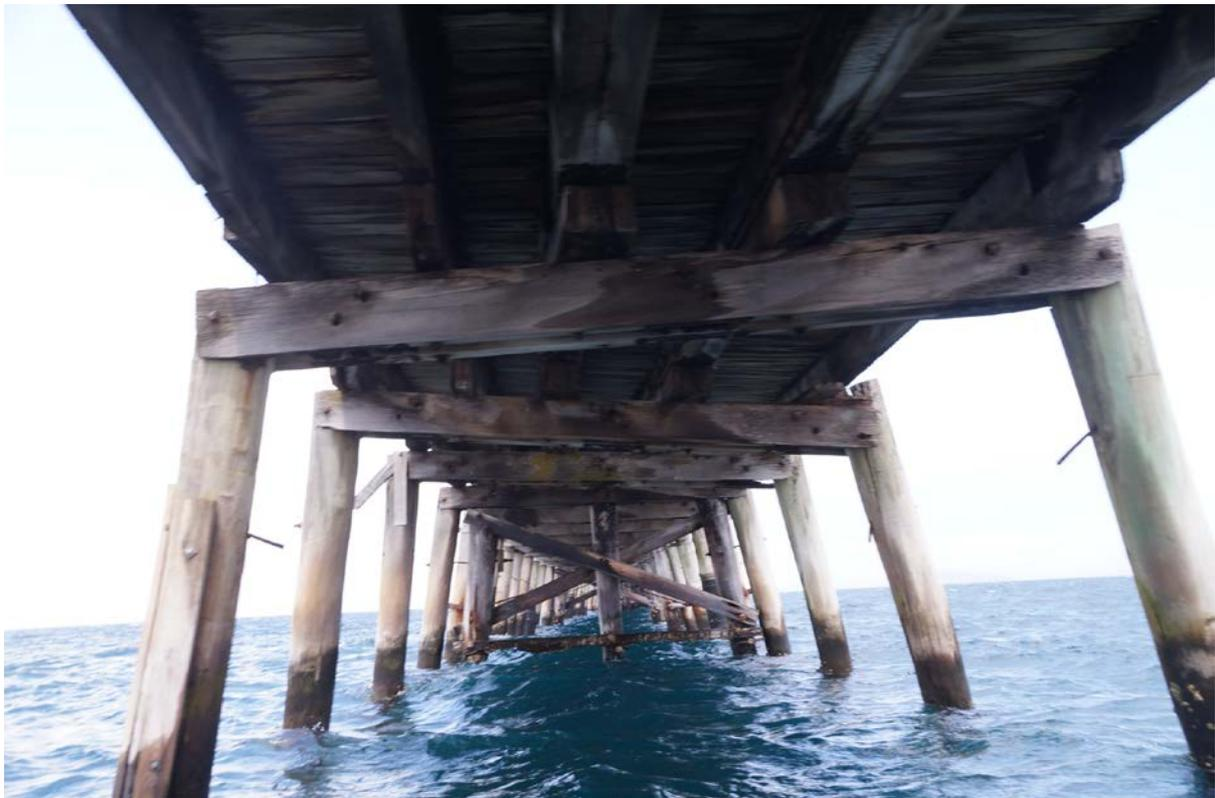
*The pile on the left hand side, which already has a splint applied from previous repairs has completely failed and is no longer supporting the deck. The half cap at the front of the photo has collapsed to the north and the next two half caps have collapsed to the south, making the deck twist.*
