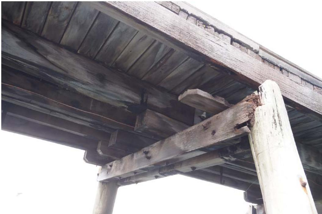
*The corbel has split and fallen away and the stringer is no longer supported by the pile underneath.*
