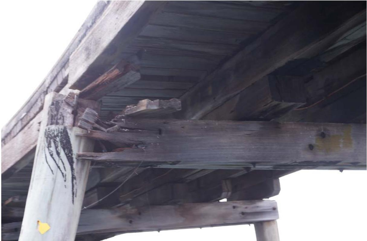
*The red wood exposed is indicative of recent failure in the half cap and corbel, highlighting that the jetty is twisting and creating new damage.*
