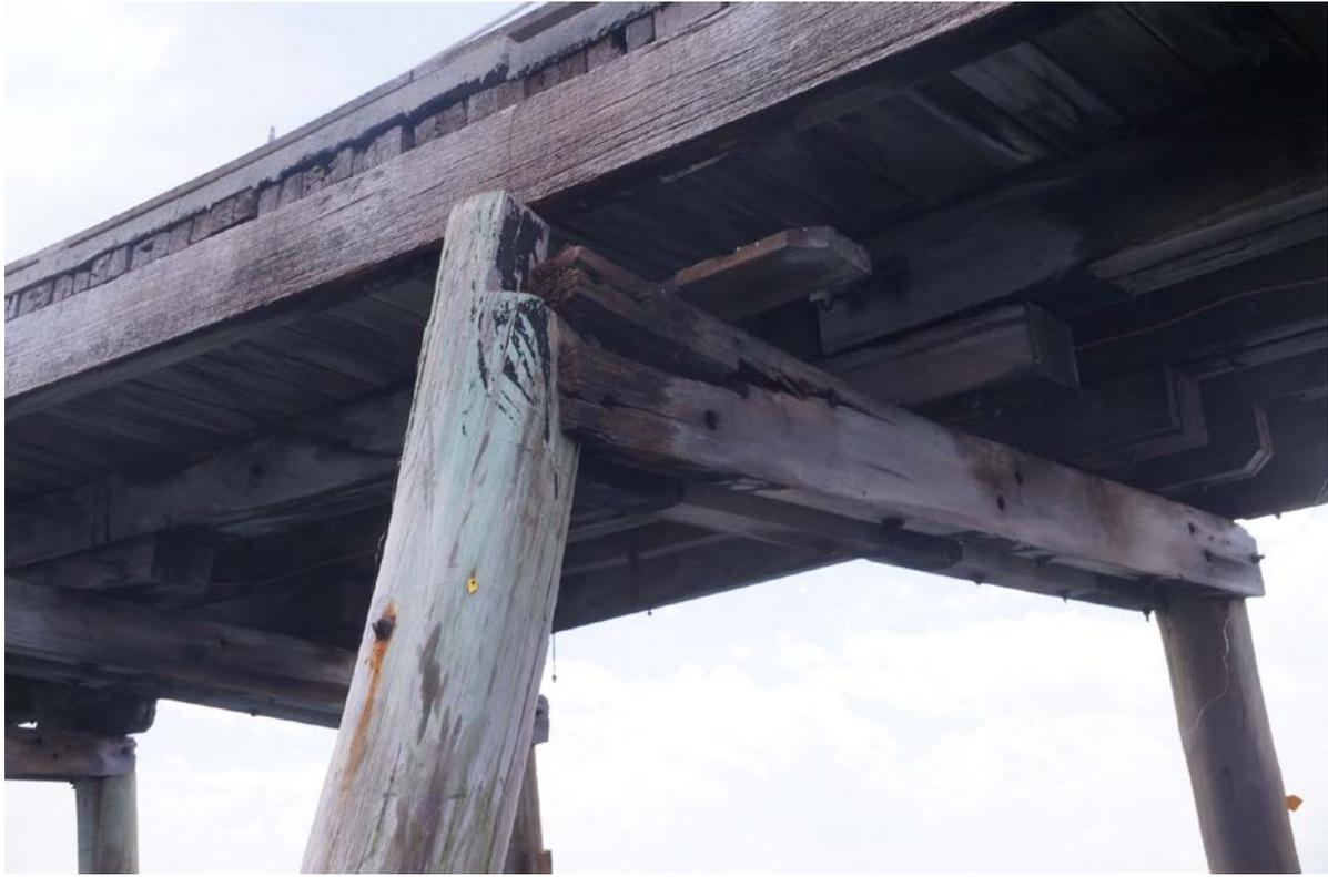
*Both the corbel and the half cap have split and been crushed. The longitudinal stringers, which are the main elements that support the deck are no longer supported by the half cap. This damage has accelerated since December 2015 and is causing the deck to sag.*
