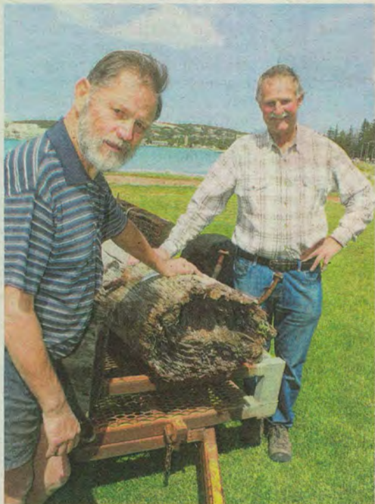
Dilapidated: John Bridges and John Hart with a rotten pylon.
