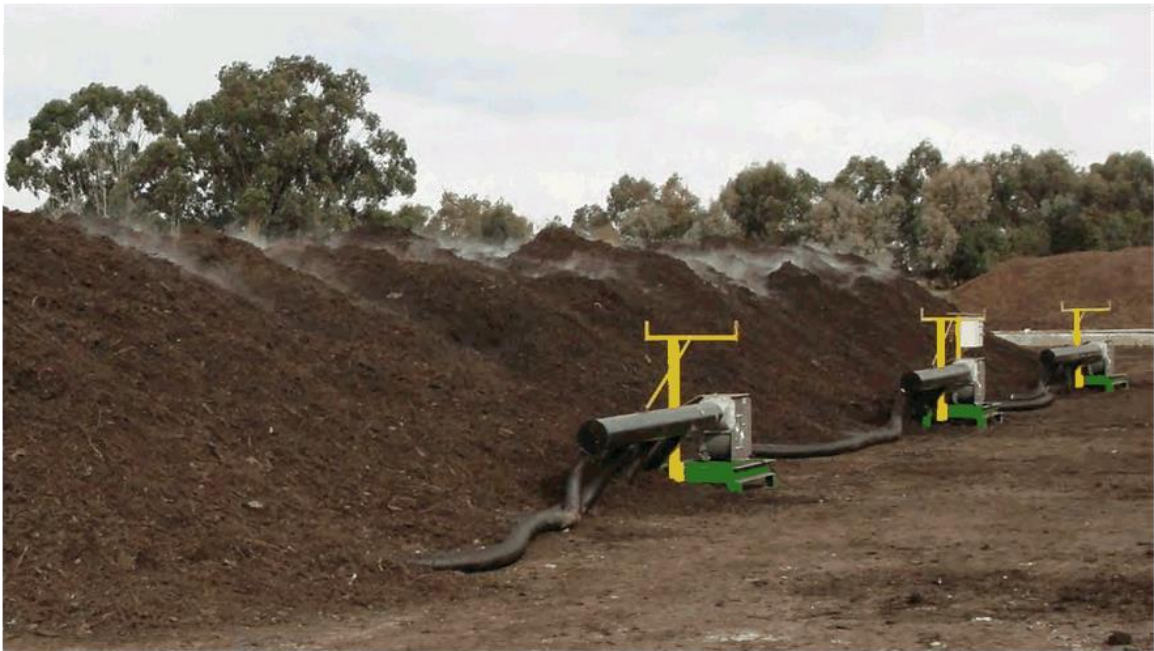
Figure 5.4 Aerated floor composting set up
