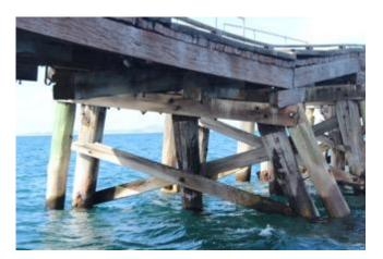
Figure 1 Pile Group 66 (missing) & 67 07/04/18
