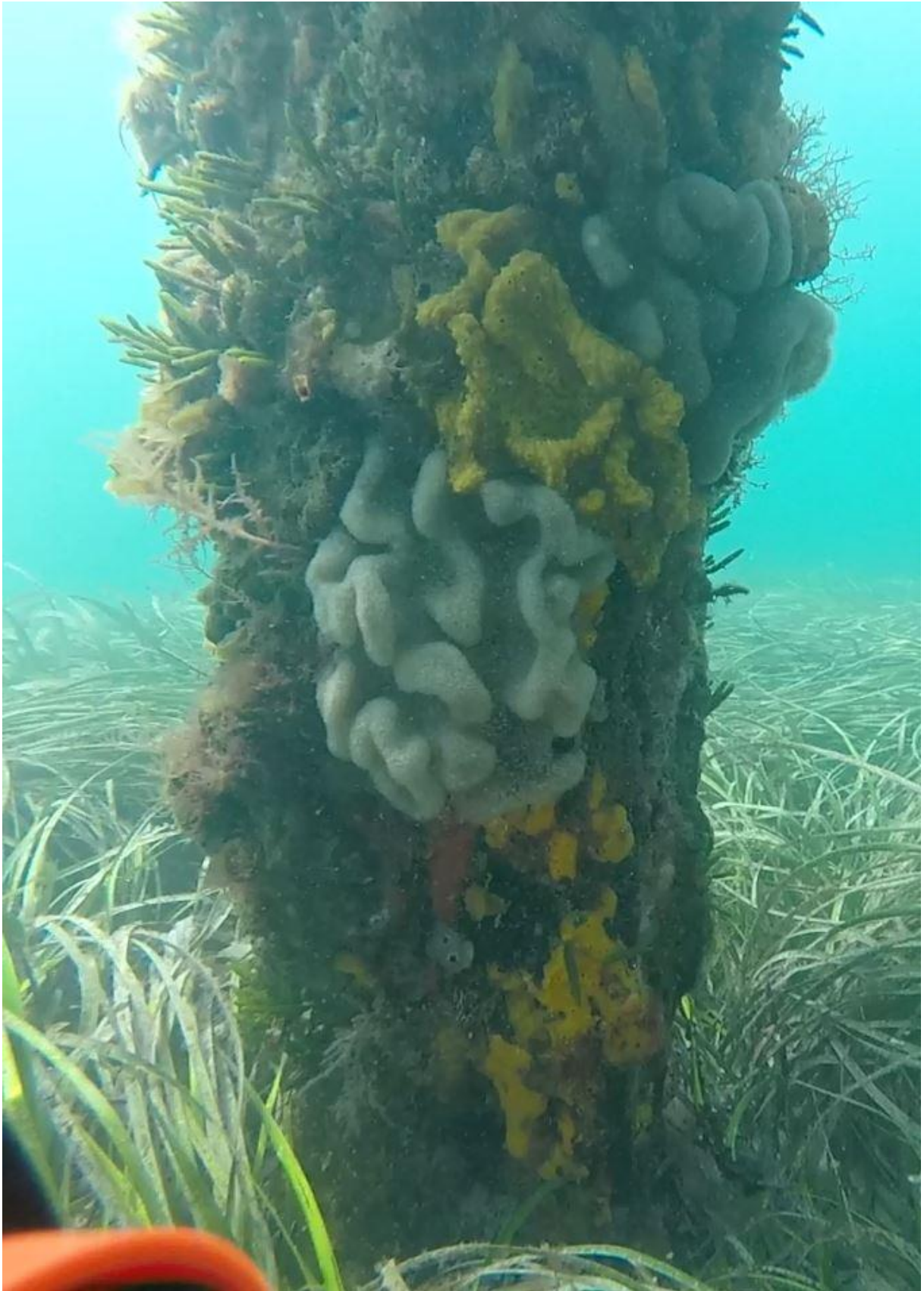
Figure 3-1: 54 North 11/11/15 – Severe necking at base (prior to failure identified 17/11/15)
