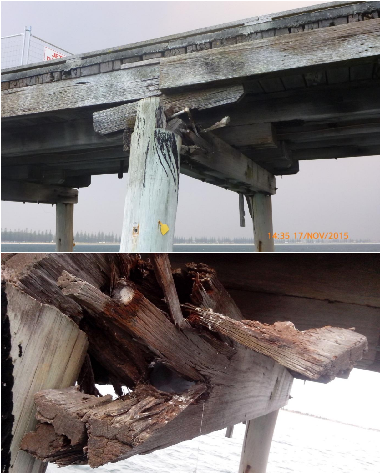
Figure 3-13: 95 Southeast (Top-17/11/15, Bottom 30/11/15) – Crushing failure of half caps
