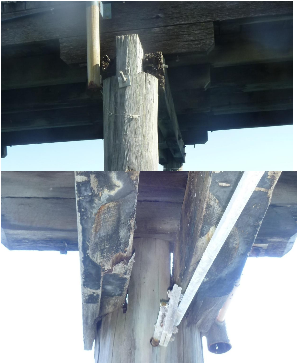
Figure 3-15: 36 North 17/11/15 – Crushing of both half caps
