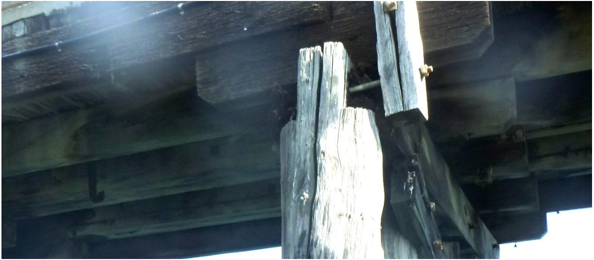
Figure 3-16: 37 North 17/11/15 – Crushing of both half caps
