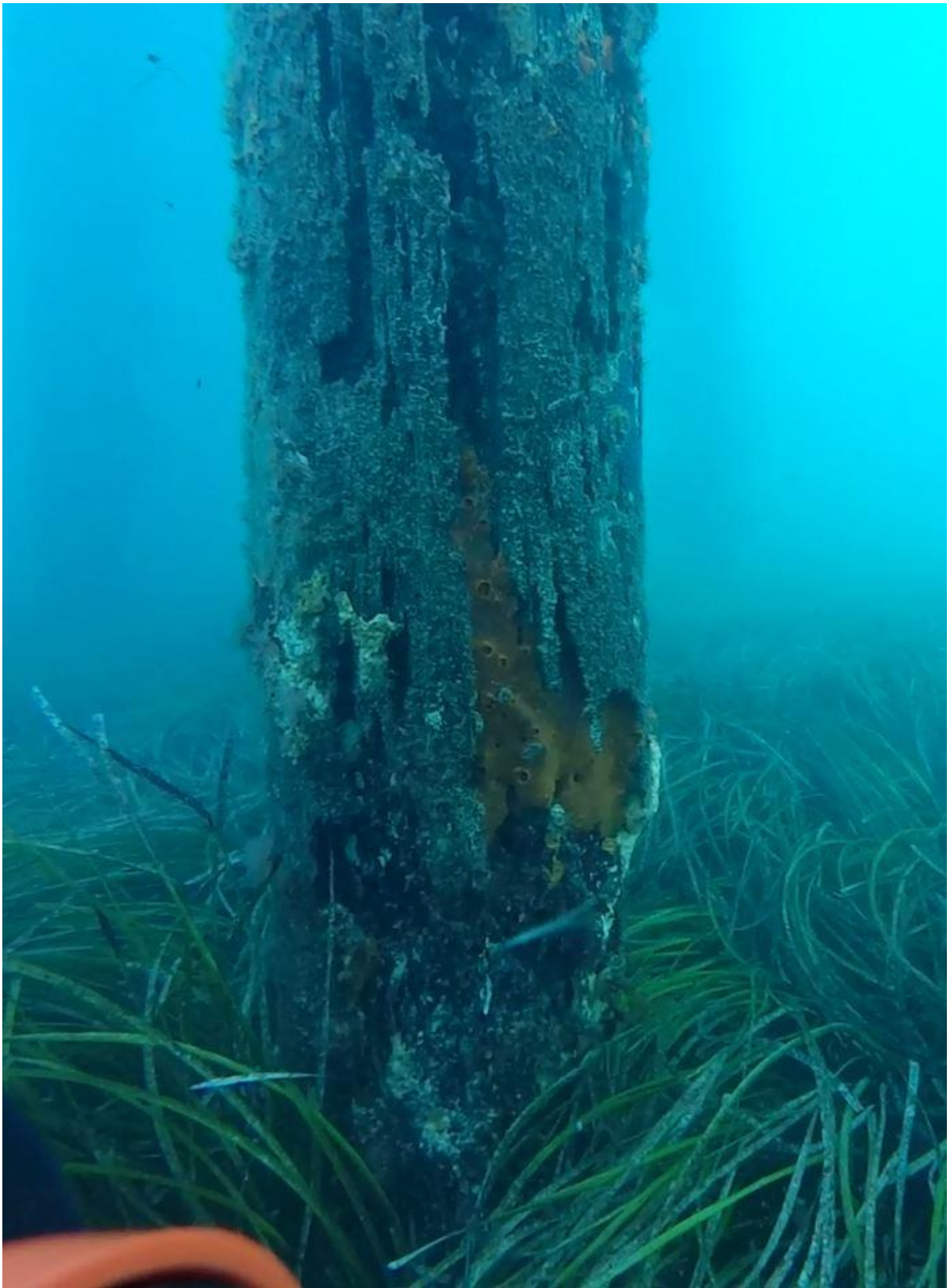
Figure 3-11: 112 North 11/11/15 – Severe section loss at base
