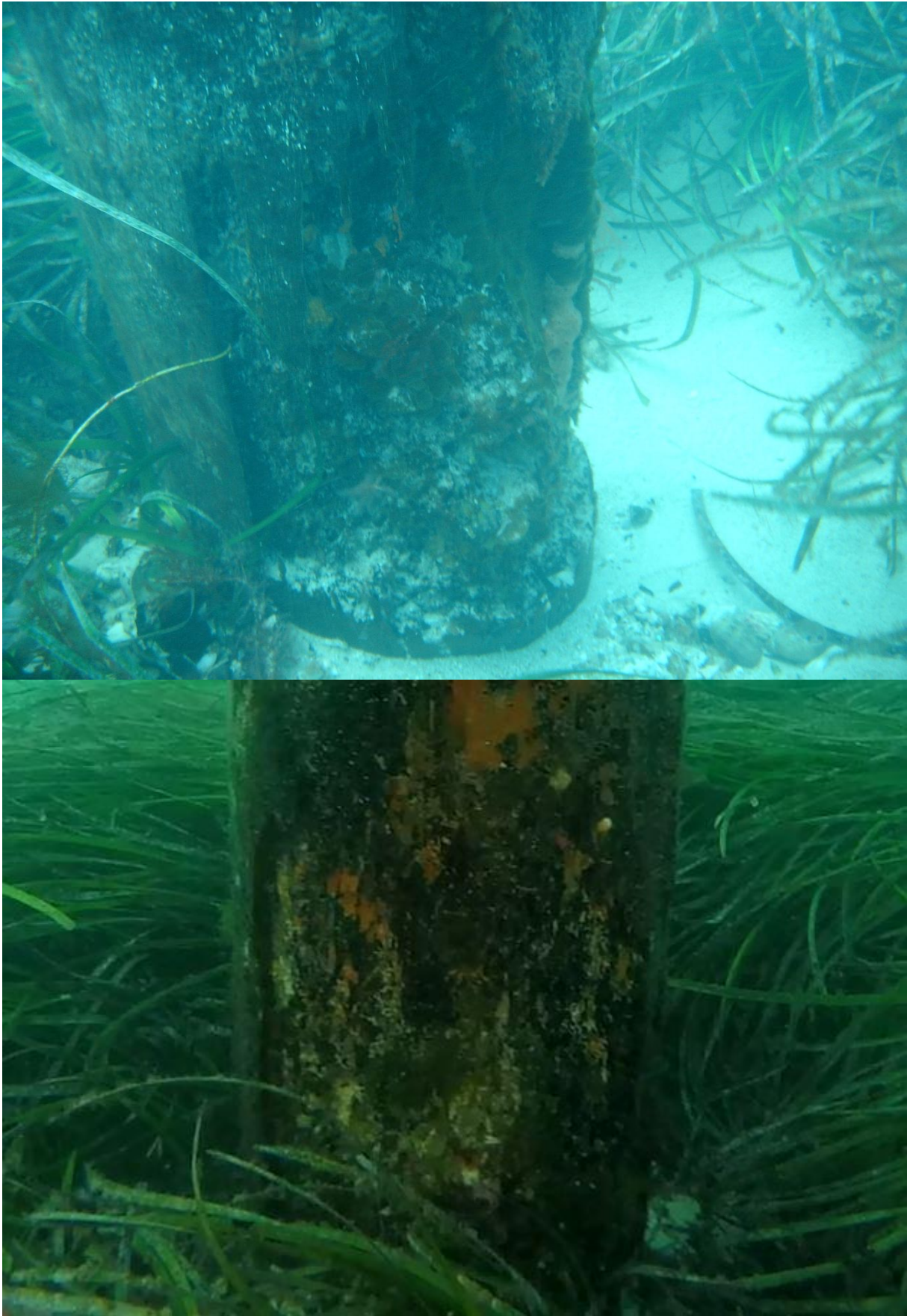
Figure 3-9: 91 North (Top-3/8/13, Bottom-11/11/15) – Severe section loss at base
