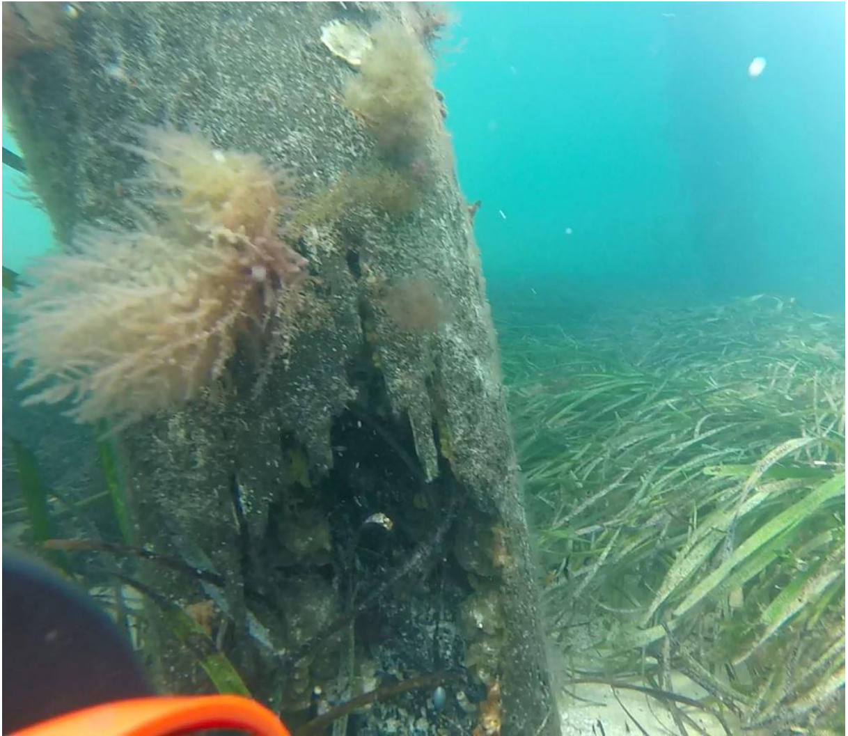
Figure 3-4: 58 South 11/11/15 – Severe section loss at base
