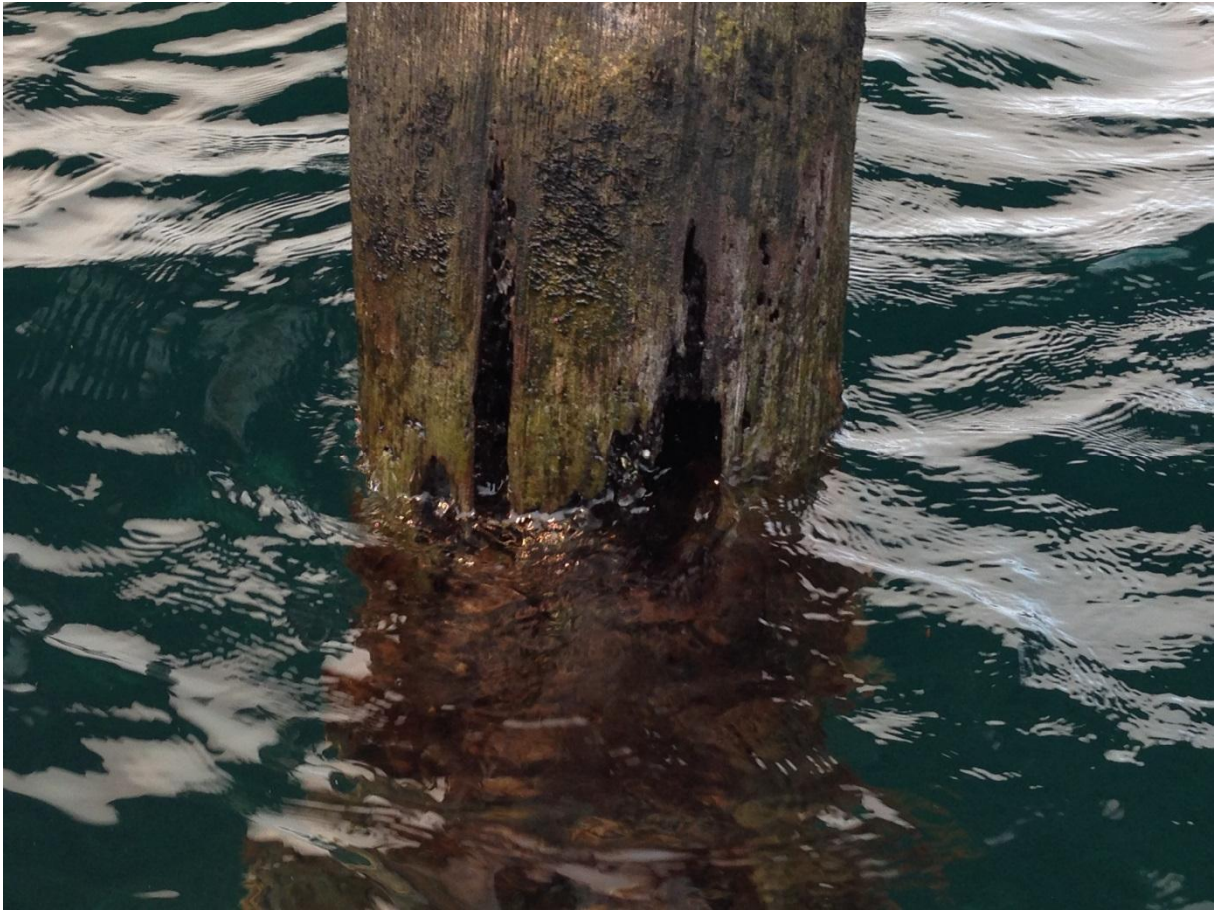
Figure 3-7: 71 South 17/11/15 – Severe section loss at surface (surface inspected only)
