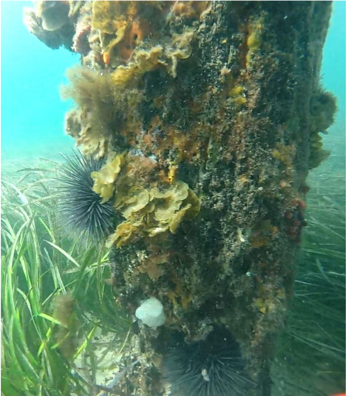
Figure 3-5: 66 North 11/11/15 – Severe section loss at base
