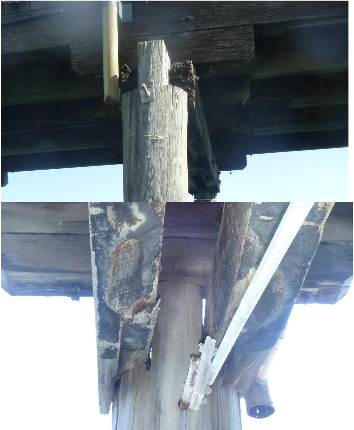
Figure 3-15: 36 North 17/11/15 – Crushing of both half caps
