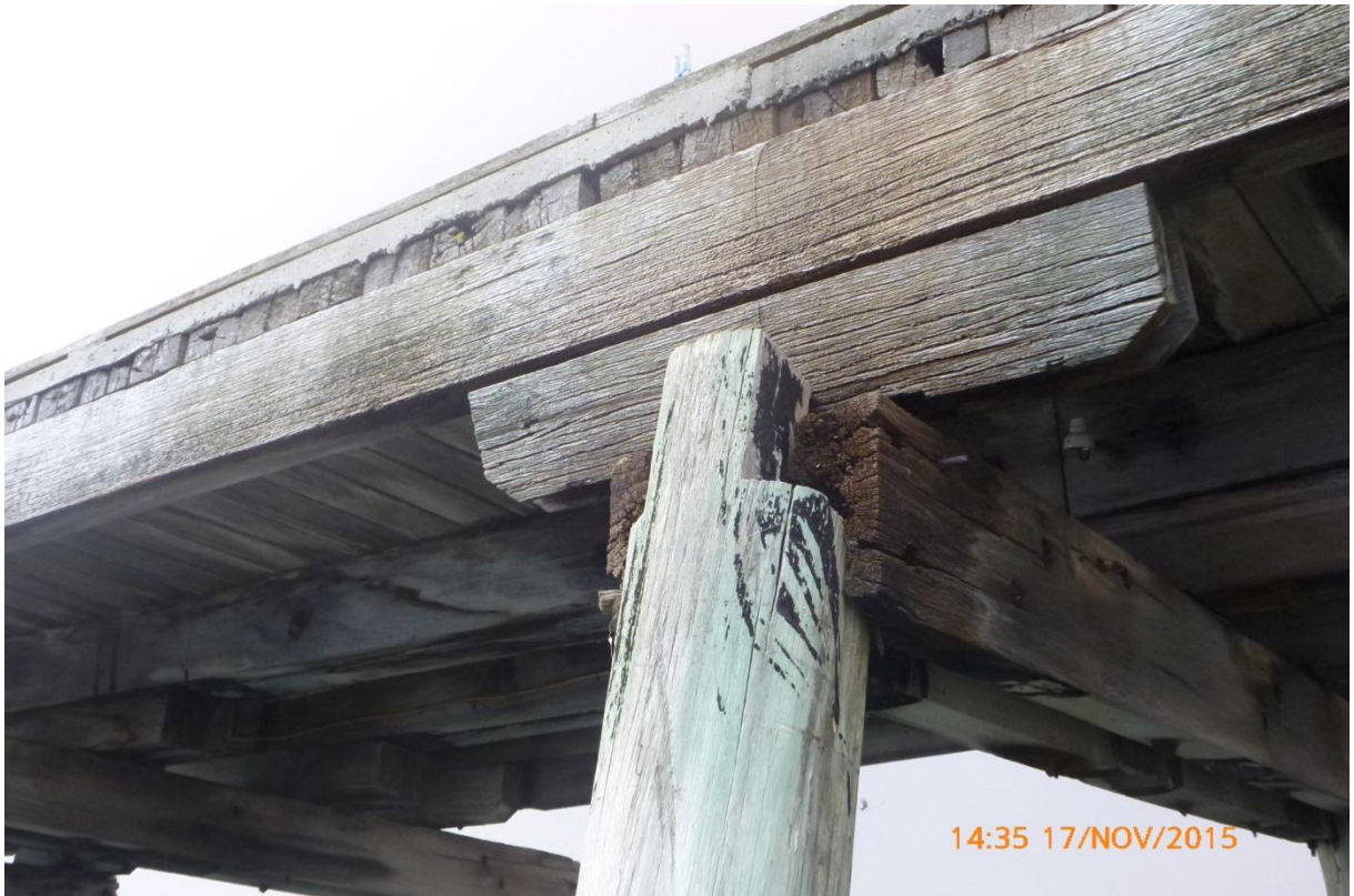
Figure 3-22: 94 South 17/11/15 – Crushing of both half caps
