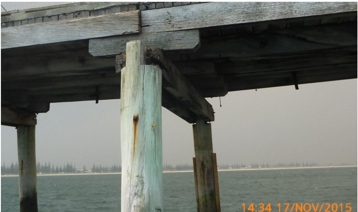
Figure 3-21: 93 South 17/11/15 – Crushing of both half caps
