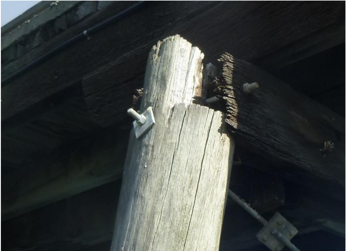
Figure 3-14: 35 North West 17/11/15 – Crushing of both half caps
