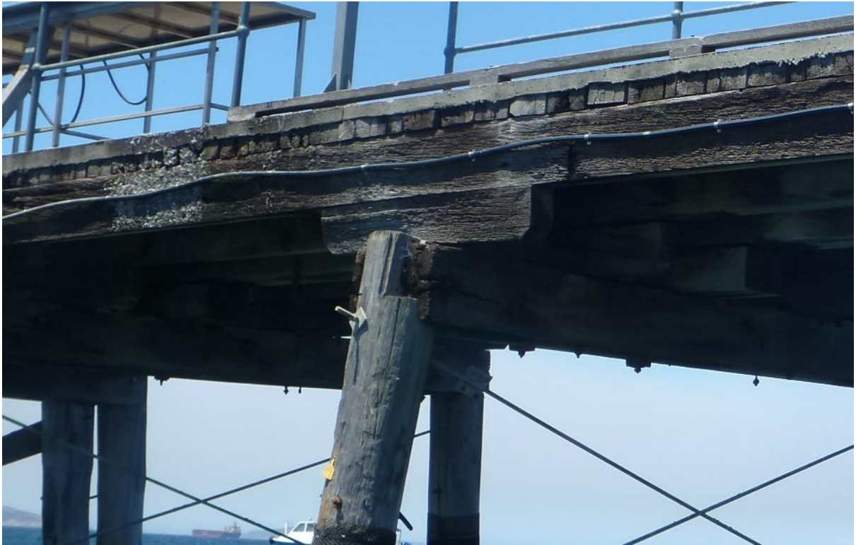
Figure 3-20: 43 North 17/11/15 – Crushing of both half caps
