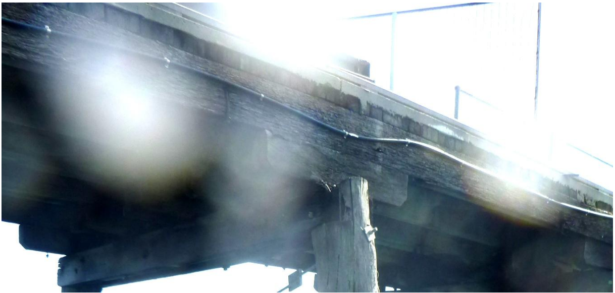
Figure 3-17: 38 North 17/11/15 – Crushing of both half caps
