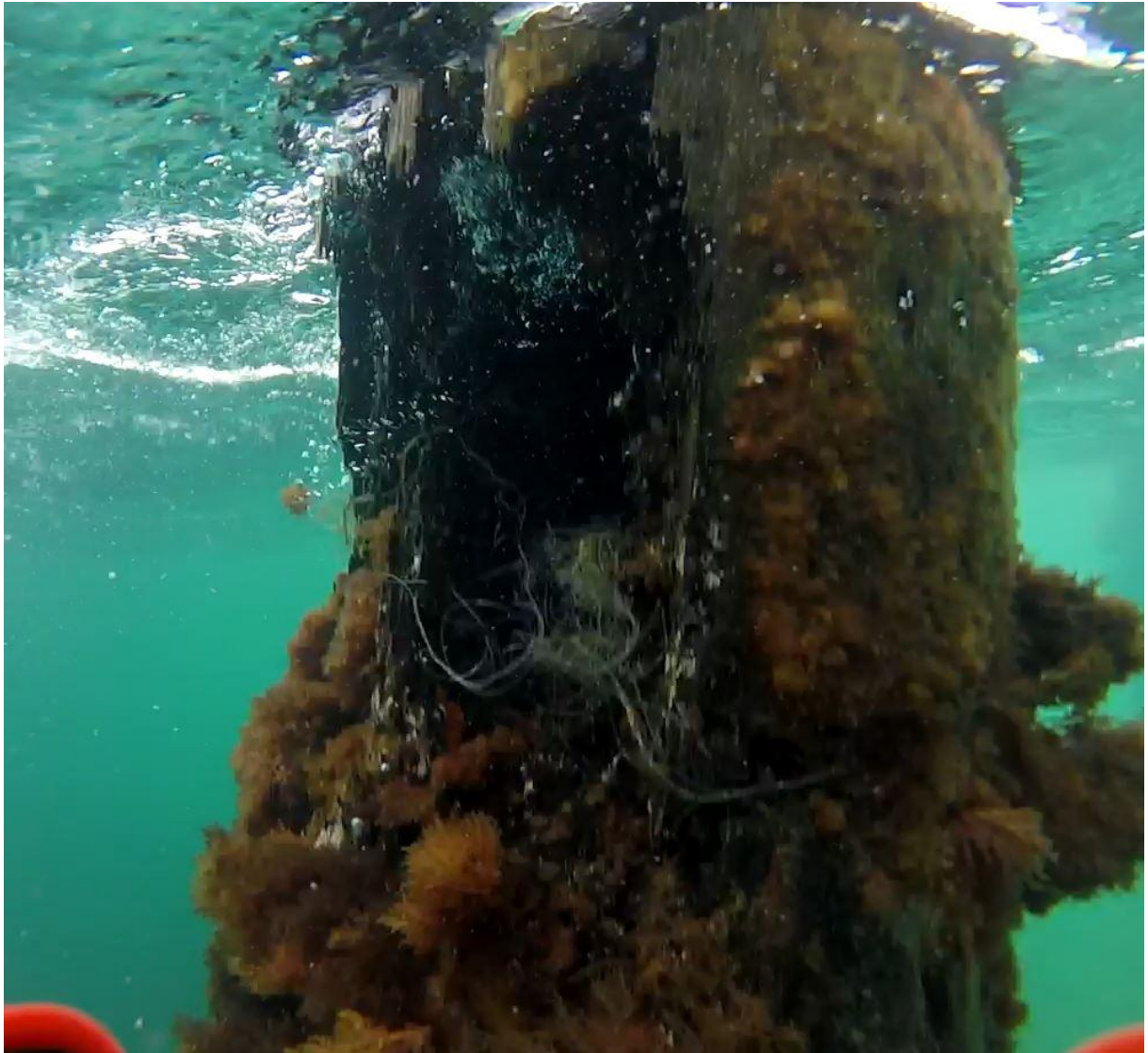
Figure 3-3: 53 South 11/11/15 – Severe section loss at surface
