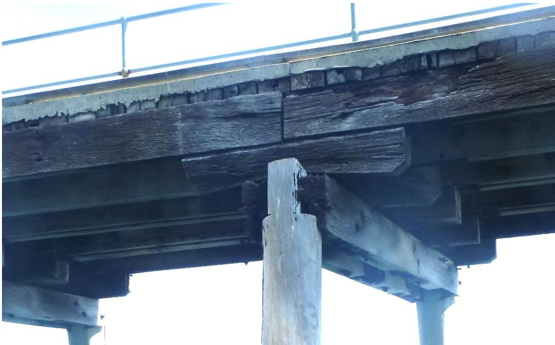
Figure 3-23: 133 North 17/11/15 – Crushing of both half caps
