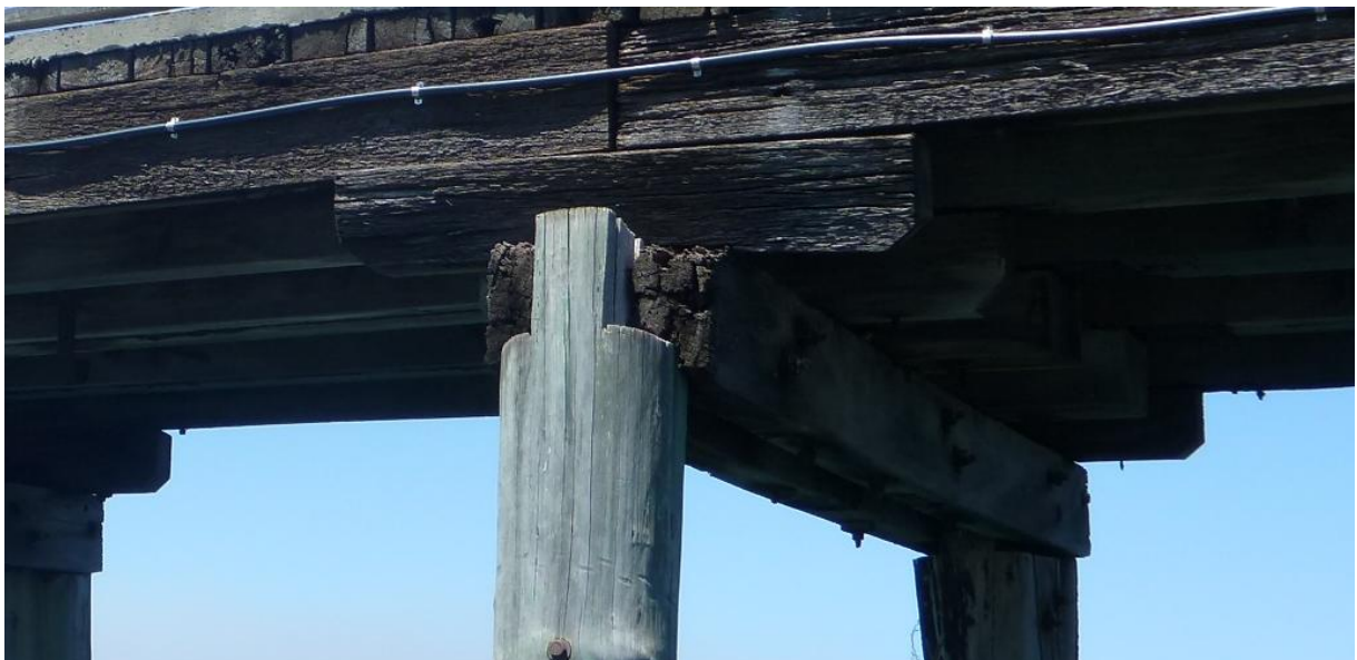
Figure 3-19: 43 North 17/11/15 – Crushing of both half caps
