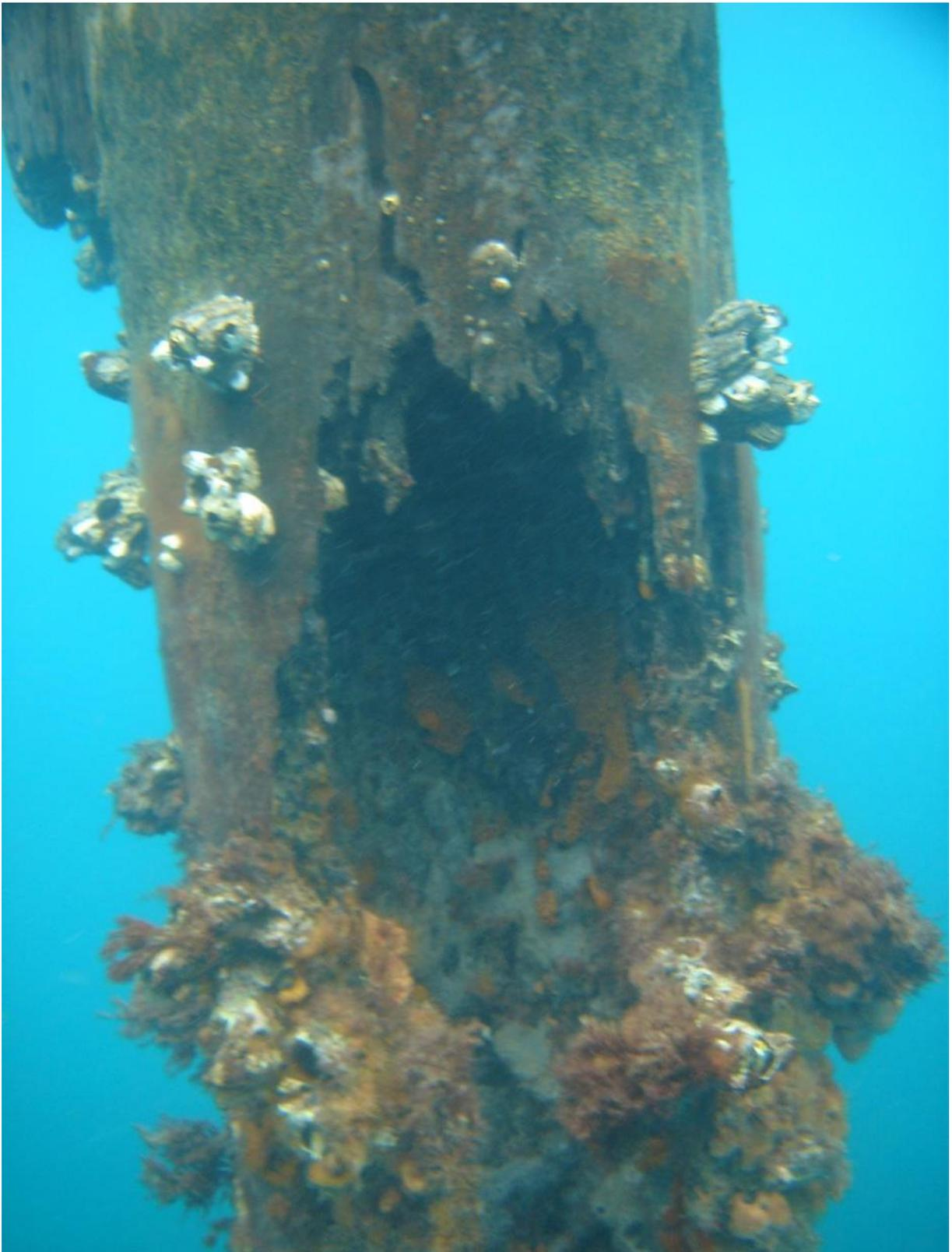
Pile 106 South has suffered significant visible section loss. There is likely to be further section loss due to Teredo worm that is not visible.
