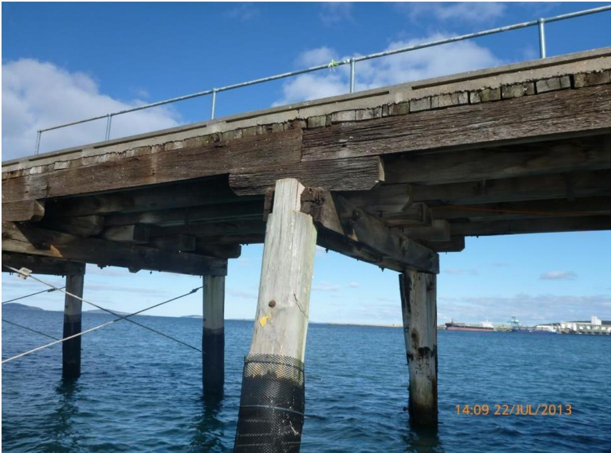
The end distance on the half cap to pile bolt connection is insufficient, and with the weathering to the half caps, the connection is no longer effective. In addition, the rot to the northwestern half cap has reduced the bearing strength sufficiently for crushing to occur. The remedial should be in order of preference where possible;
