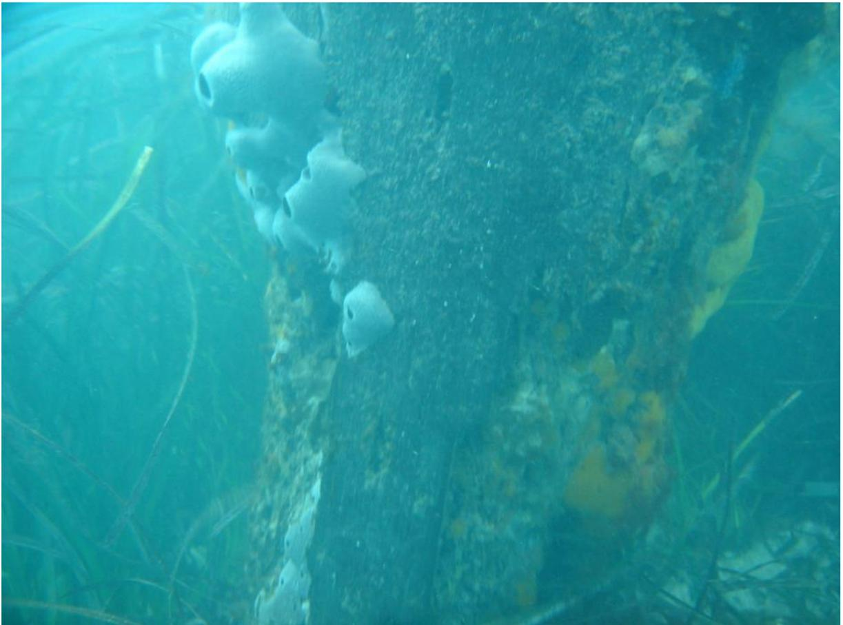
Pile 62 South has suffered significant visible section loss. There is likely to be further section loss due to Teredo worm that is not visible. A screwdriver was pushed into rotten section approximately 50mm.
