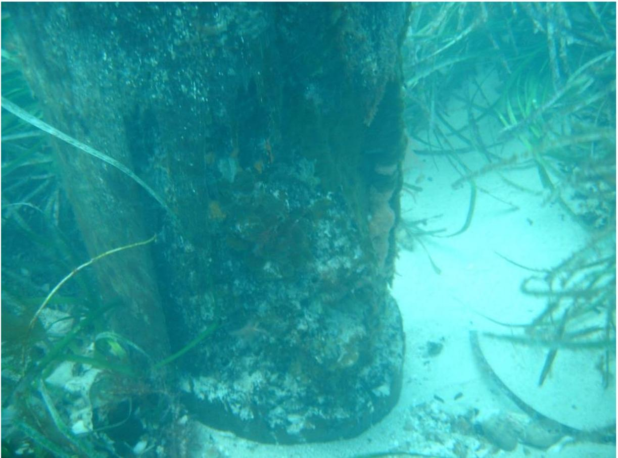
Pile 91 North has suffered significant visible section loss. There is likely to be further section loss due to Teredo worm that is not visible. Pieces of rotten timber were able to be broken off.
