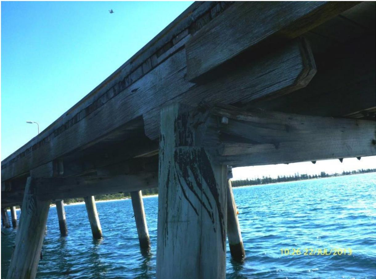
The end distance on the half cap to pile bolt connection is insufficient, and with the weathering to the half caps, the connection is no longer effective. In addition, the rot to the south-eastern half cap has reduced the bearing strength sufficiently for crushing to occur. The remedial should be in order of preference where possible;
