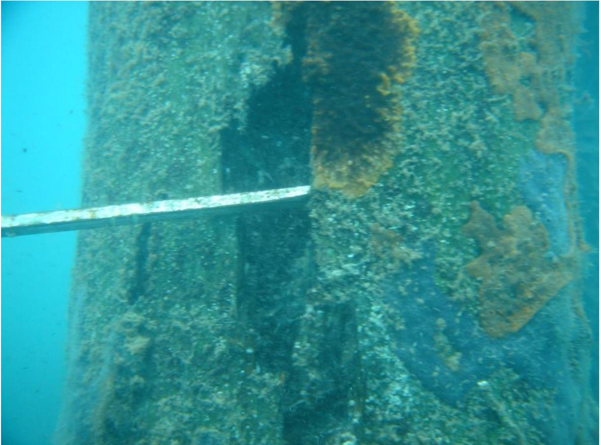
Pile 75 North has minor section loss locally a screw driver can be driven in 25mm. This pile will require remediation within 24 months, if left untreated.
