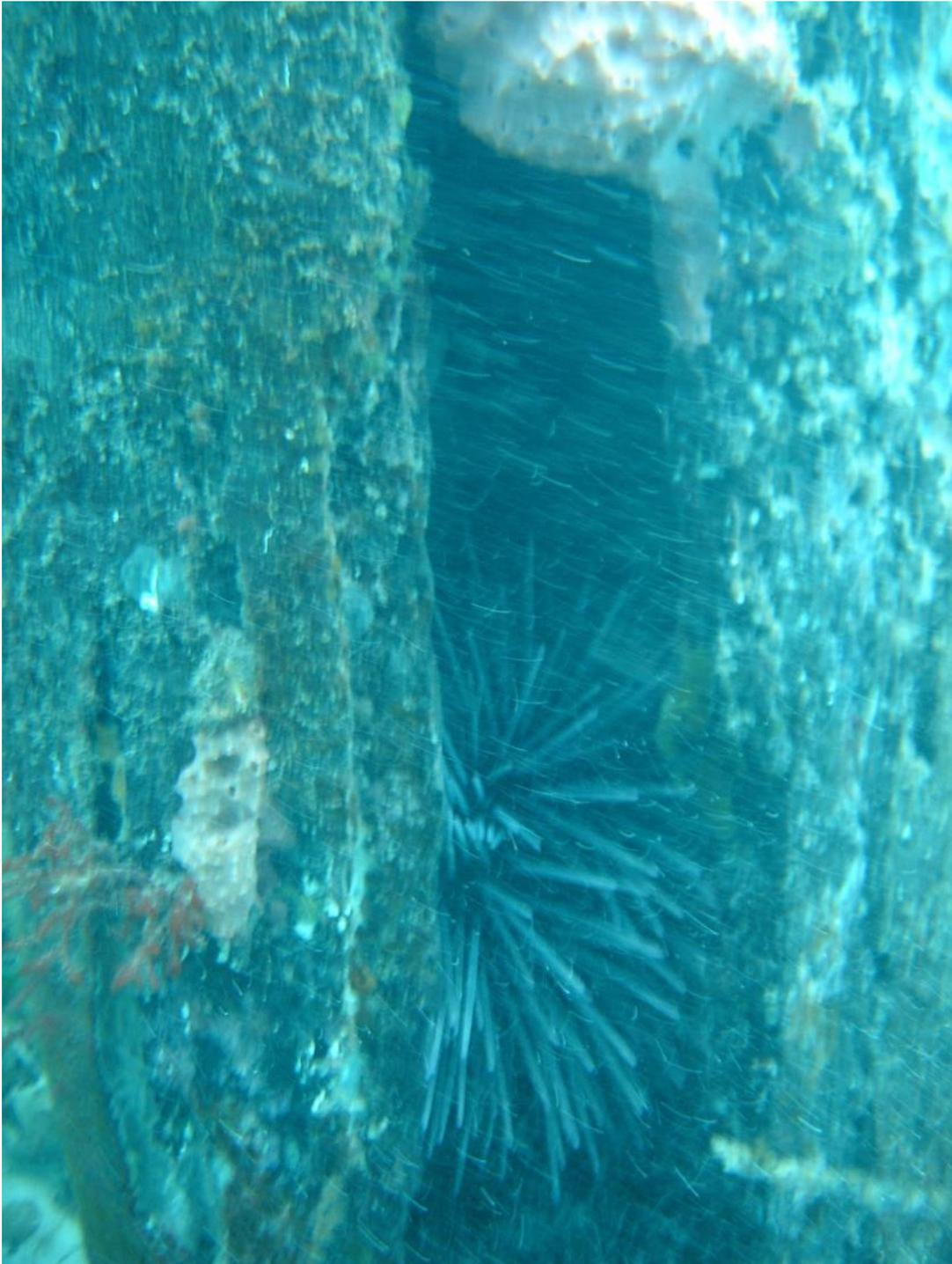
Pile 101 North has suffered significant visible section loss. Divers reported a solid centre.
