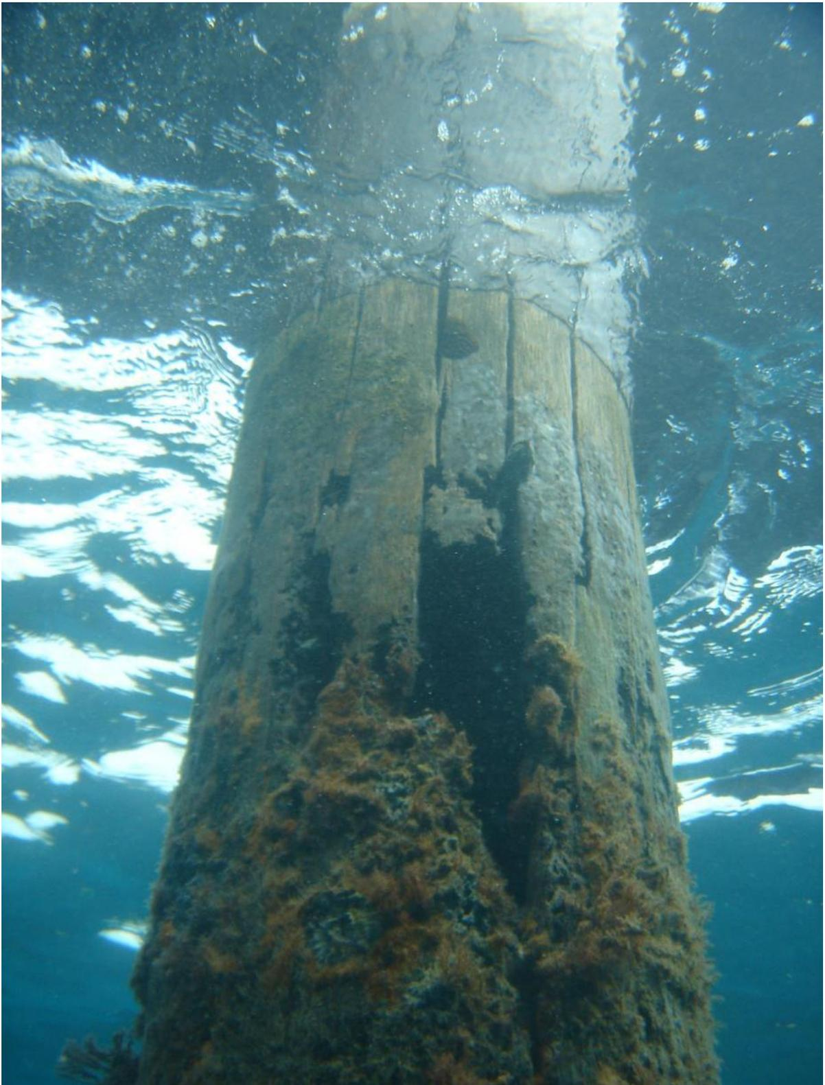
Pile 93 North was reported as having holes over its submerged length to bed level. There is likely to be significant section loss.
