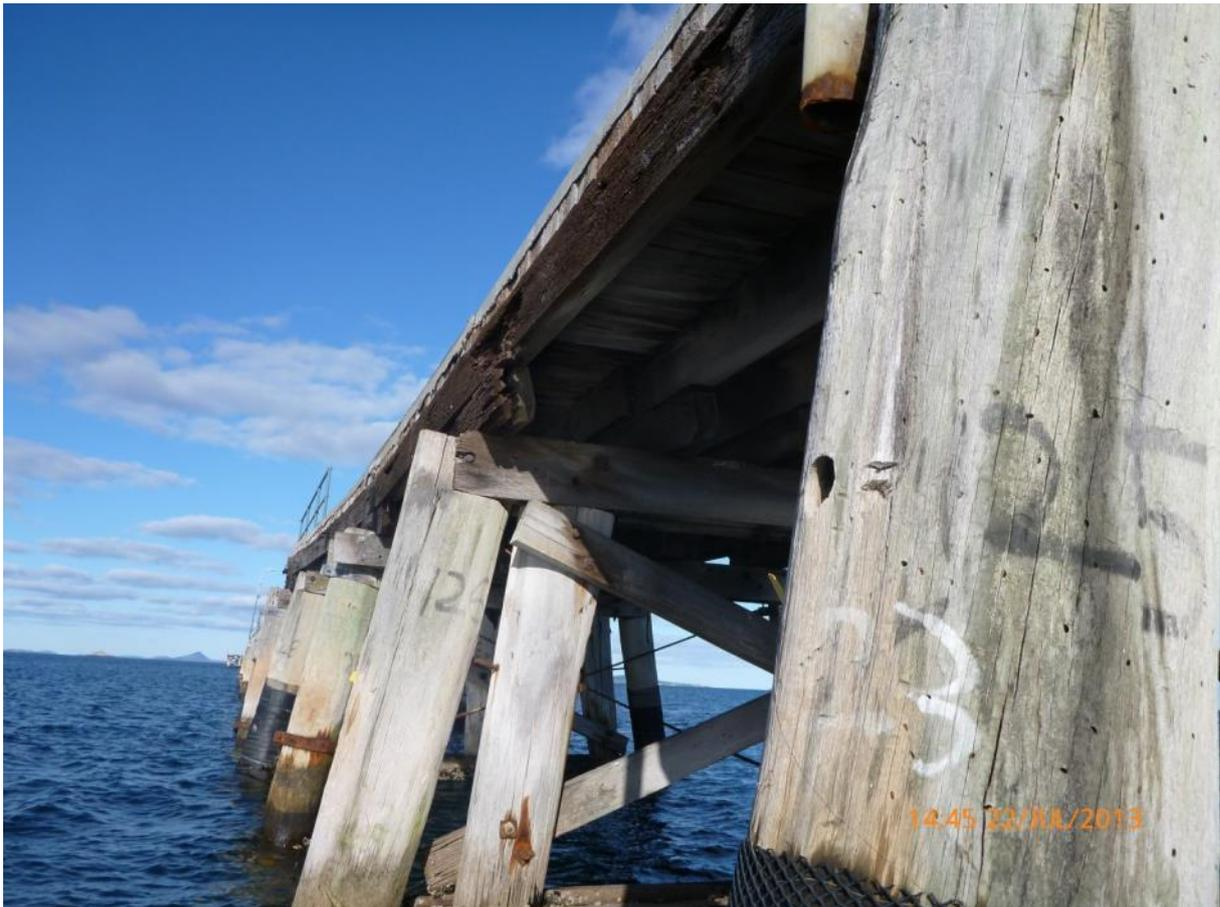
The corbel has split, has rotted and rotated about the longitudinal axis. The remedial should be in order of preference where possible;
