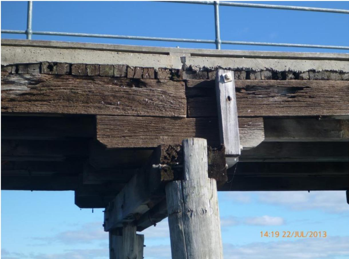
The end distance on the half cap to pile bolt connection is insufficient, and with the weathering to the half caps, the connection is no longer effective. The remedial should be in order of preference where possible;
