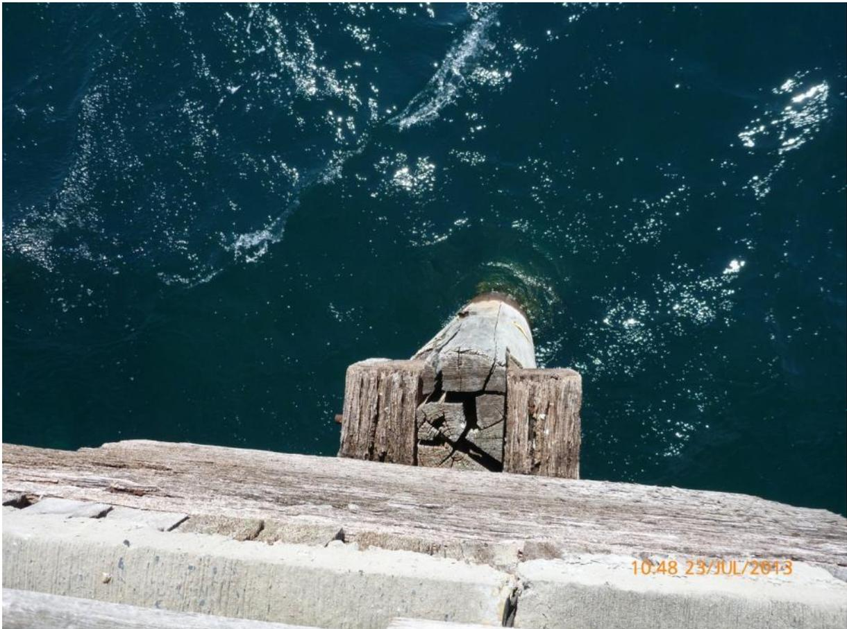
The top of the pile has split at the bolted interface with the half caps. The remedial should be in order of preference where possible;
