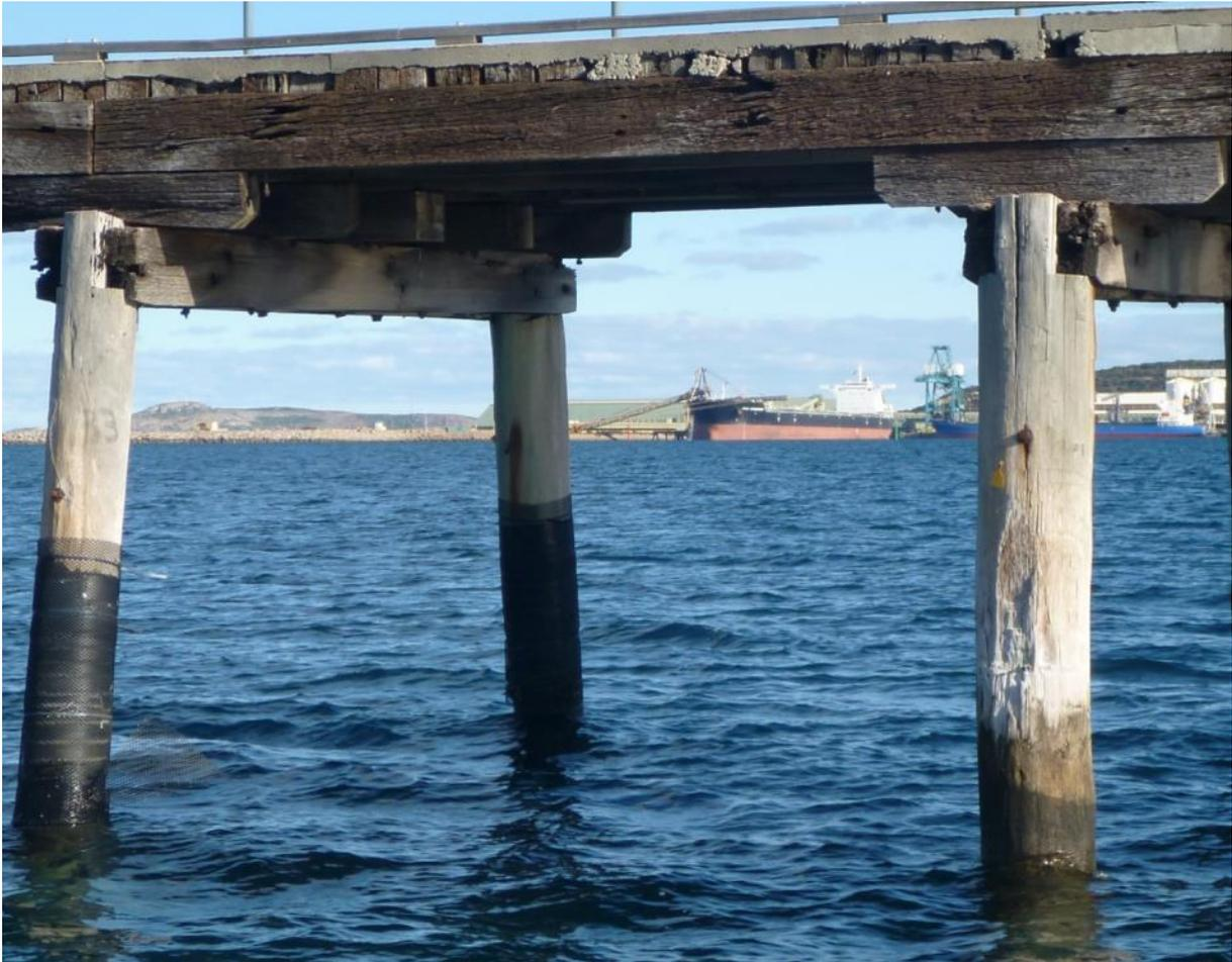
Pier 132, the north end of both half caps the pile bolt connection has insufficient end distance, and with the weathering to the half caps, the connection is no longer effective. The remedial should be in order of preference where possible;
