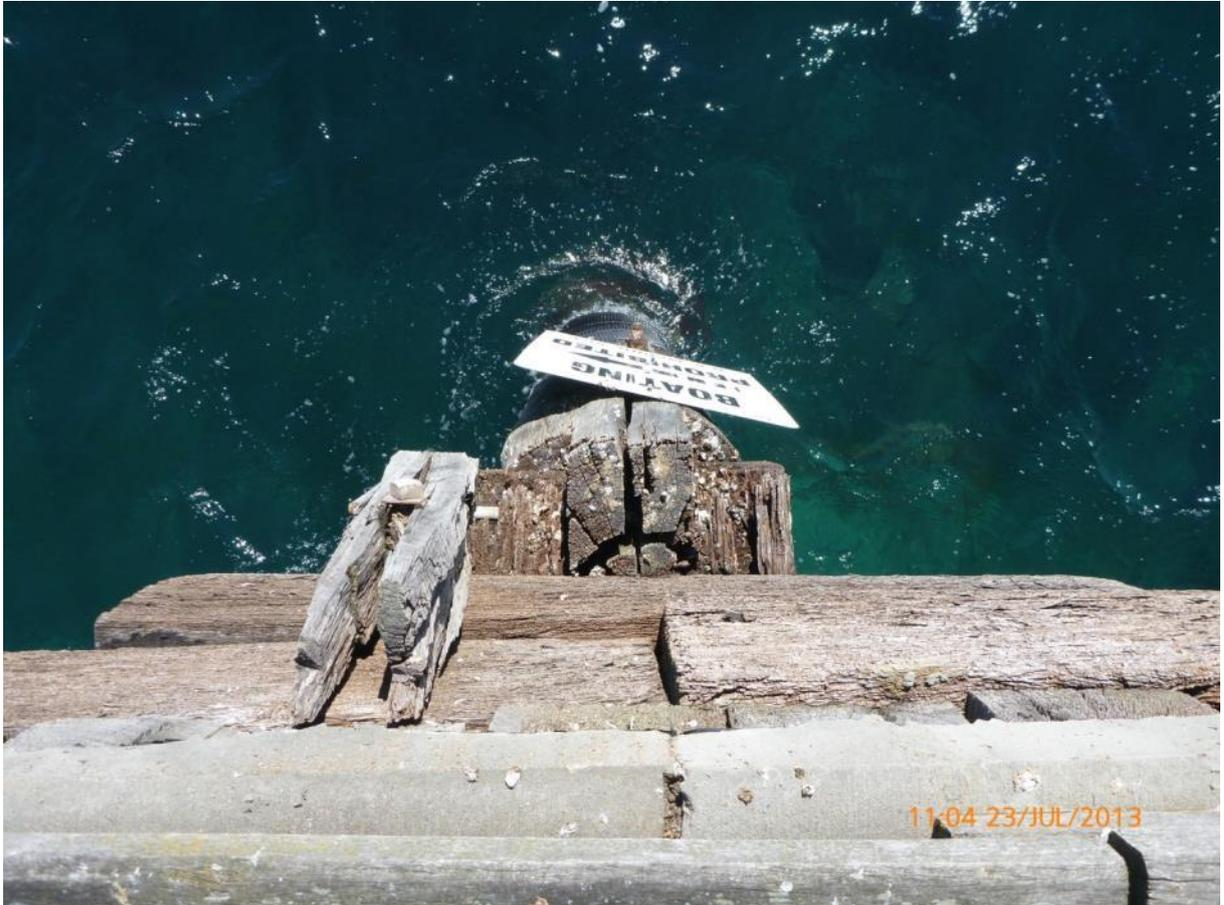
The top of the pile is split longitudinally. The remedial should be in order of preference where possible;
