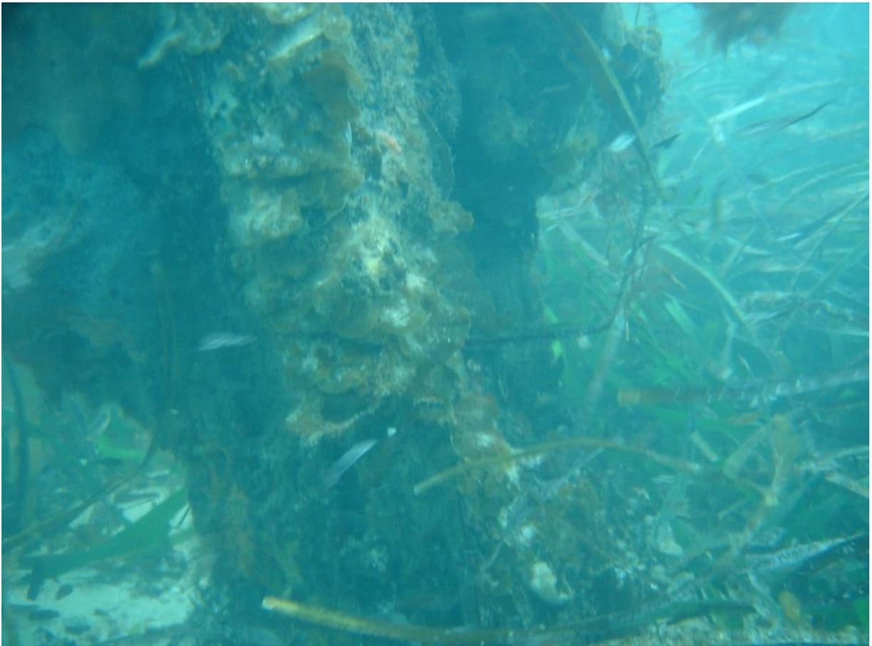
Pile 61 South has suffered visible section loss. There is likely to be further section loss due to Teredo worm that is not visible.
