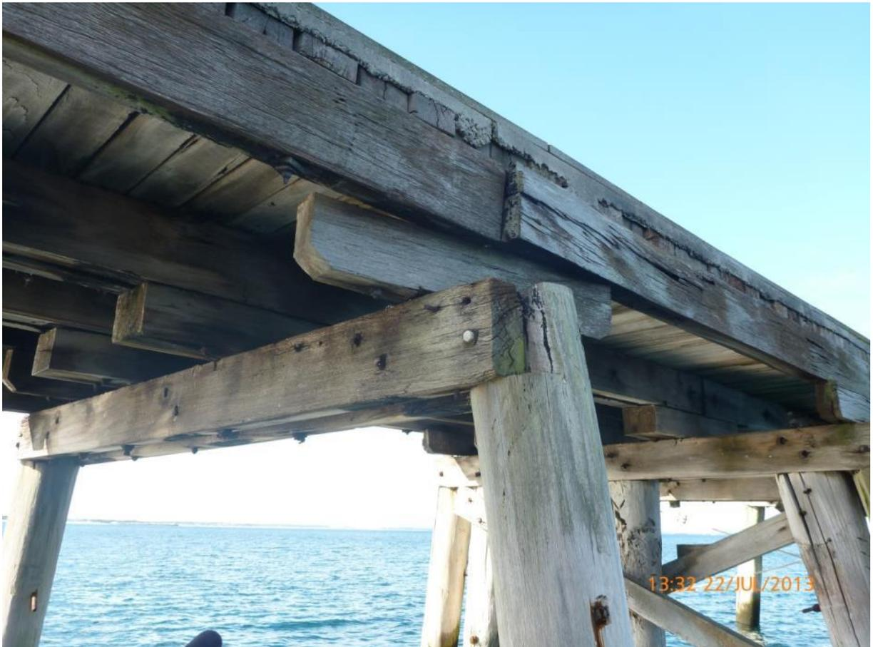
Corbel has rotated on plan. . The remedial should be in order of preference where possible;
