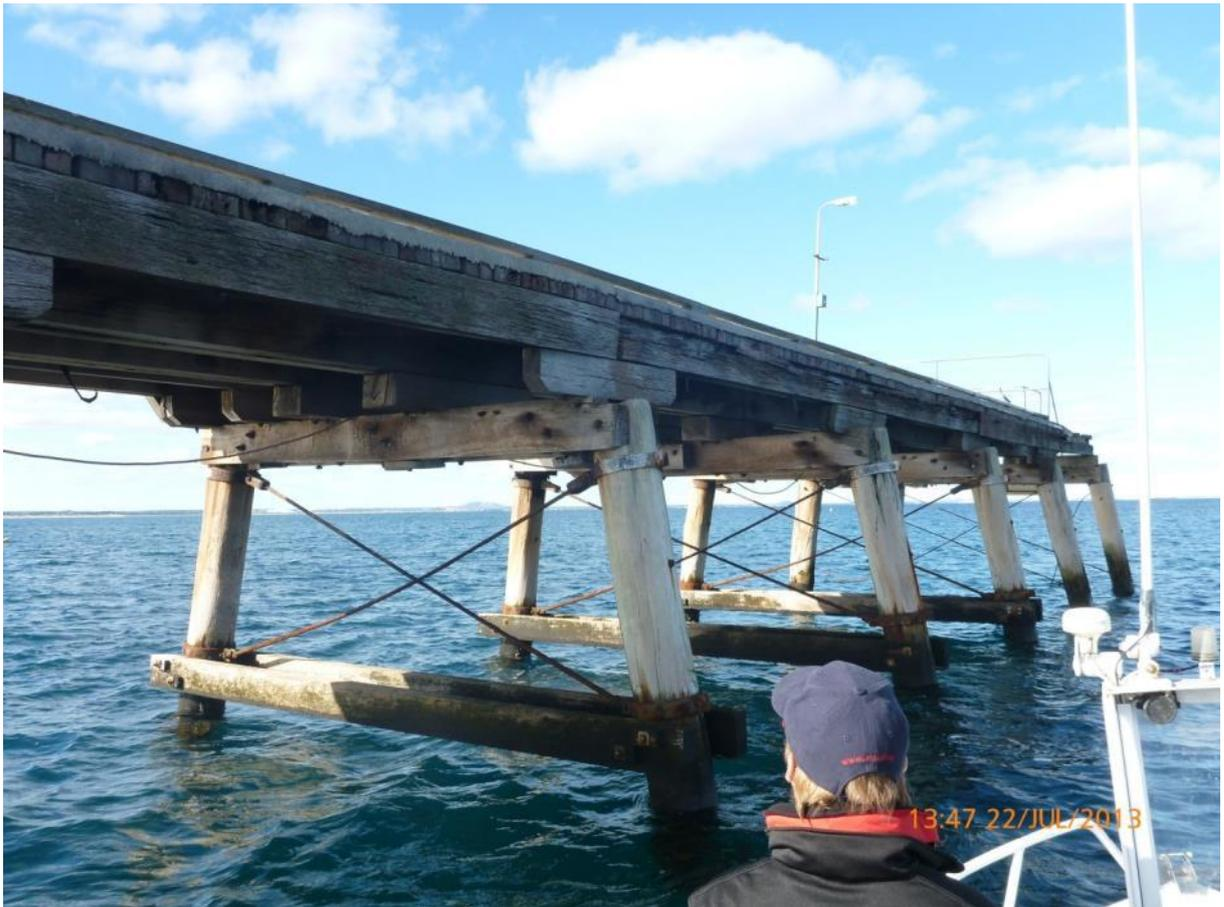
Stringer has weathered and deteriorated beyond repair. The remedial should be in order of preference where possible;
