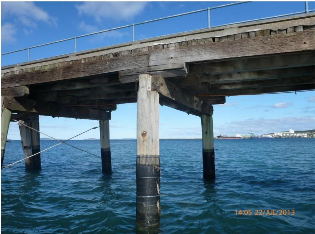
The corbel has split and crushed. The remedial should be in order of preference where possible;
