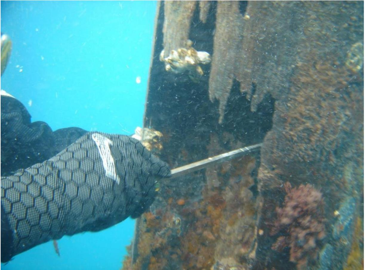
Pile 115 South has suffered very severe section loss. Divers found the affected area to be rotten and a screwdriver could be pushed into remaining section pile.
