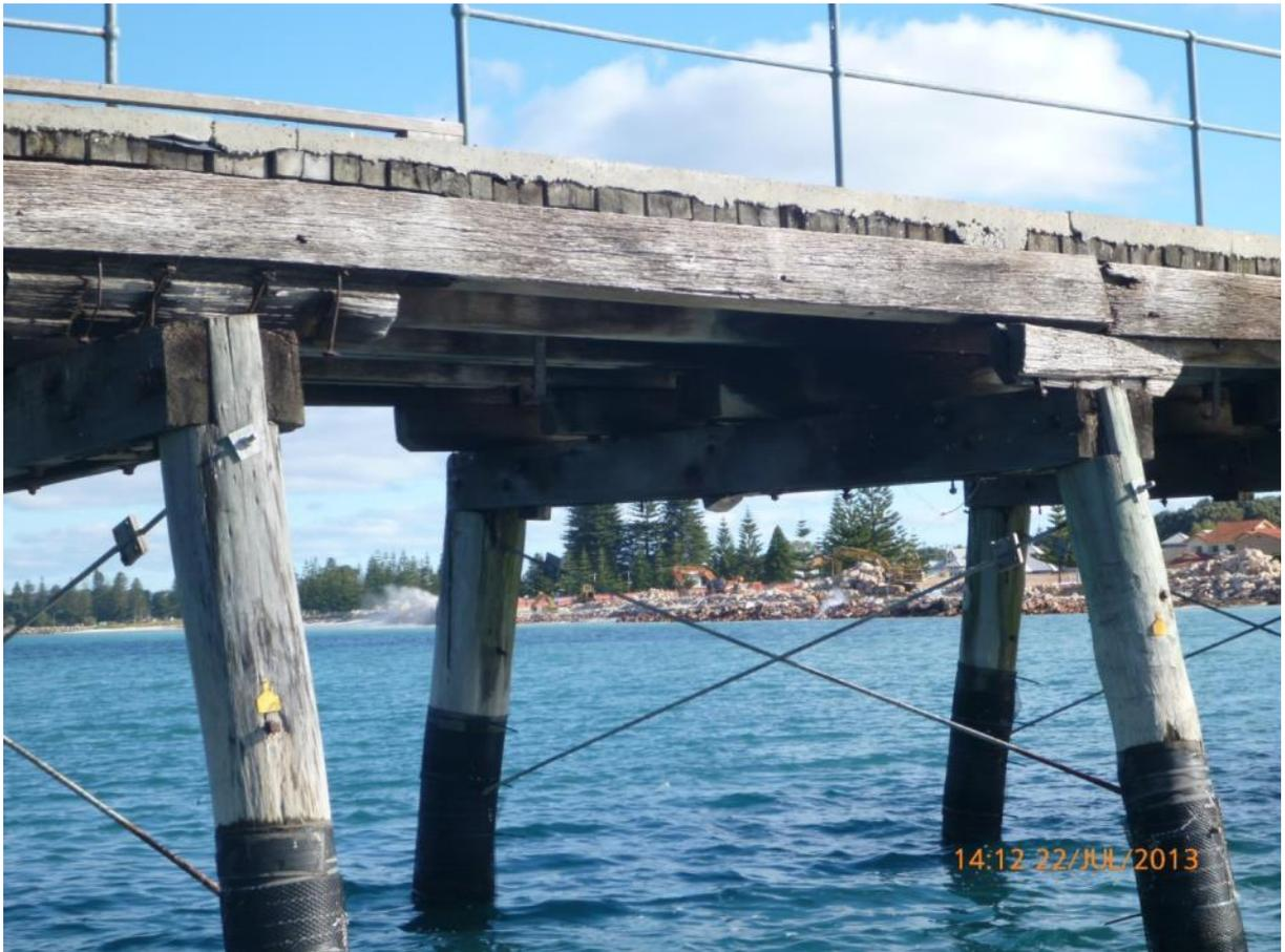
The corbels have split and rotated about the longitudinal axis. The remedial should be in order of preference where possible;
