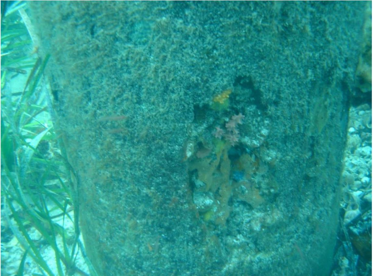
Pile 96 North has minor section loss. This pile will require remediation within 24 months, if left untreated.
