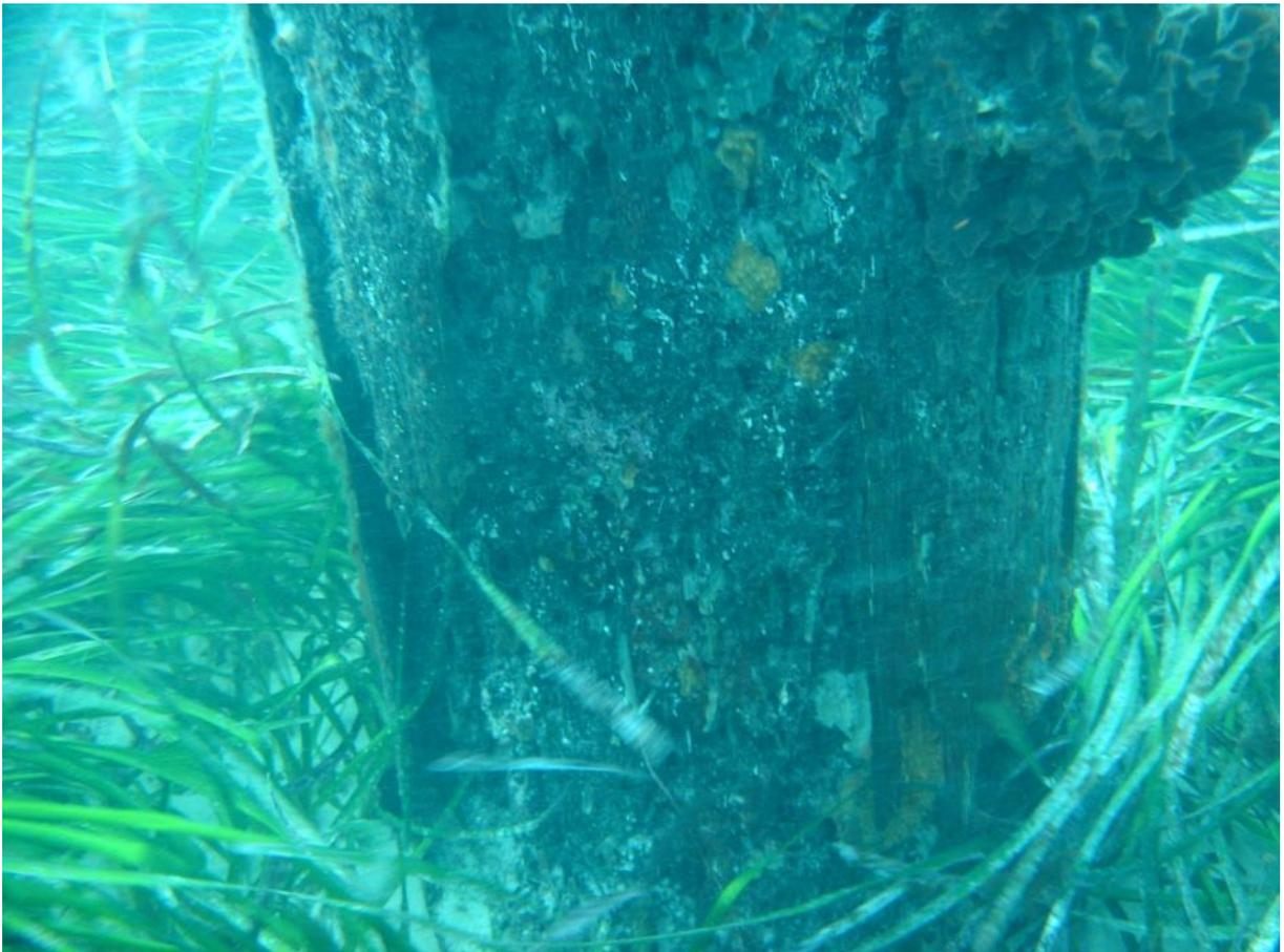
Pile 112 North has suffered some visible section loss. Divers found the affected area to be rotten and a screwdriver could be pushed approximately 40mm into pile.
