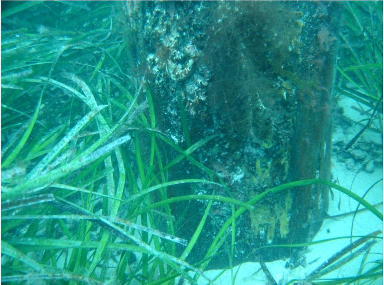
Pile 105 South has suffered significant visible section loss. Divers reported a solid centre.
