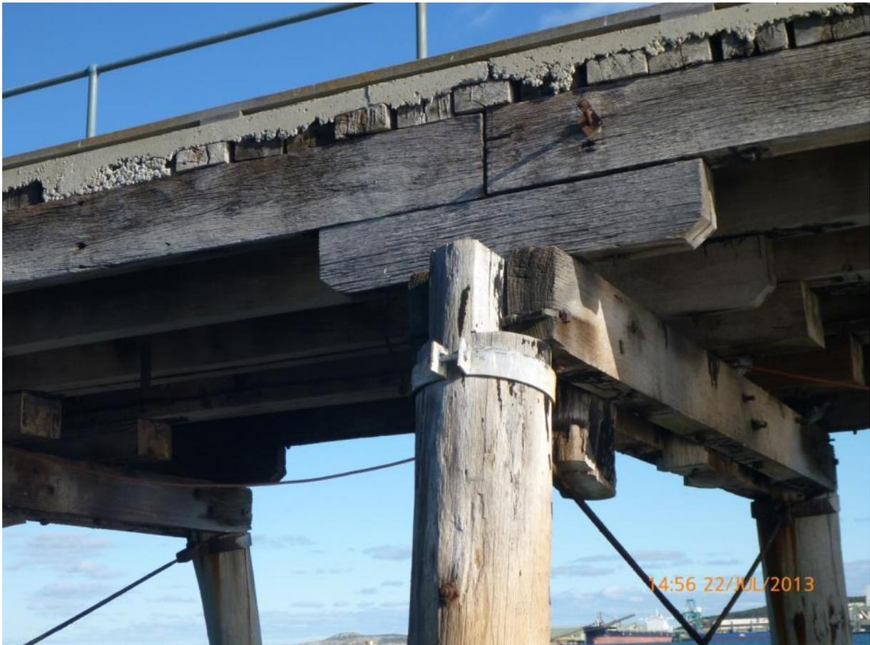
The end distance on the half cap to pile bolt connection is insufficient. There has been a shear failure of the timber suggesting that the half caps have been sliding relative to the piles. The remedial should be in order of preference where possible;
