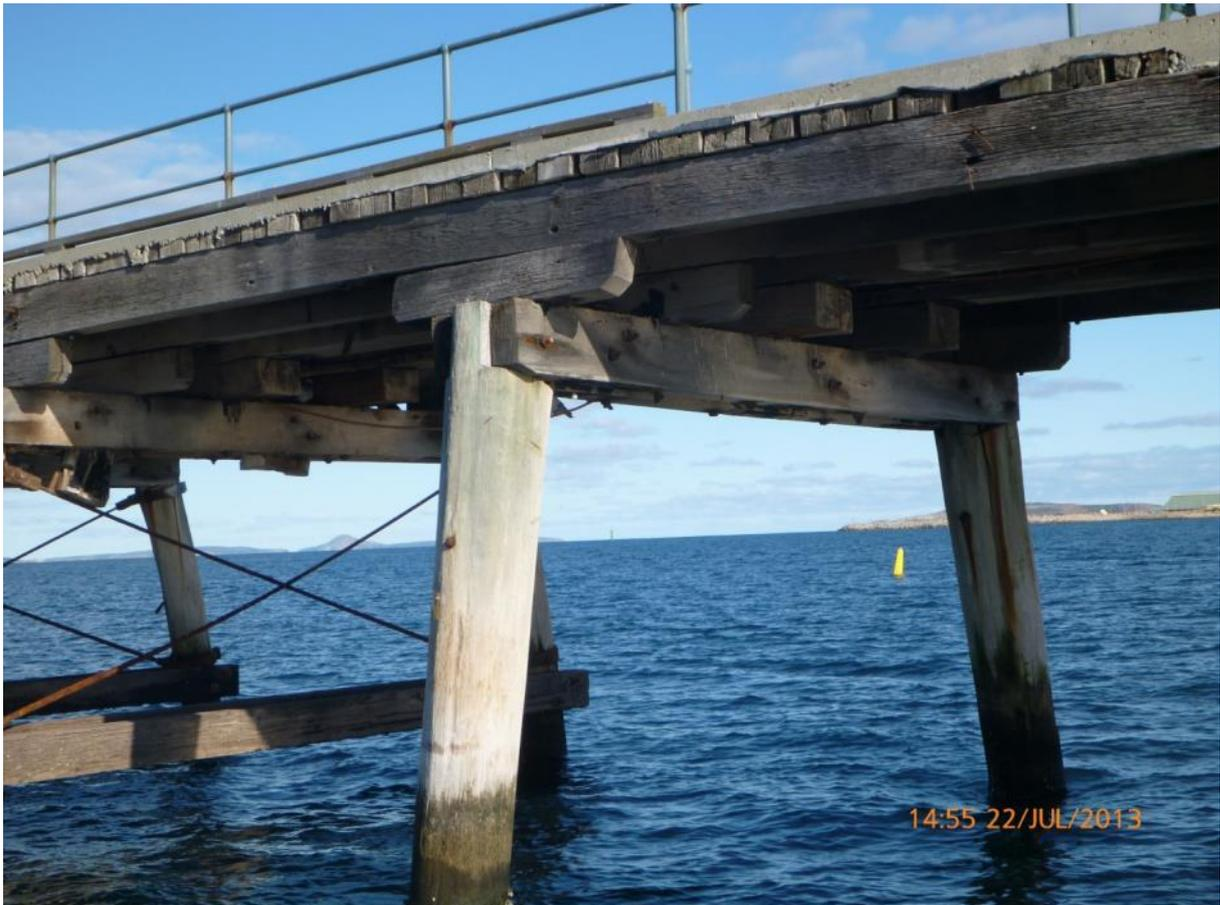
The corbel has rotated. The remedial should be in order of preference where possible;
