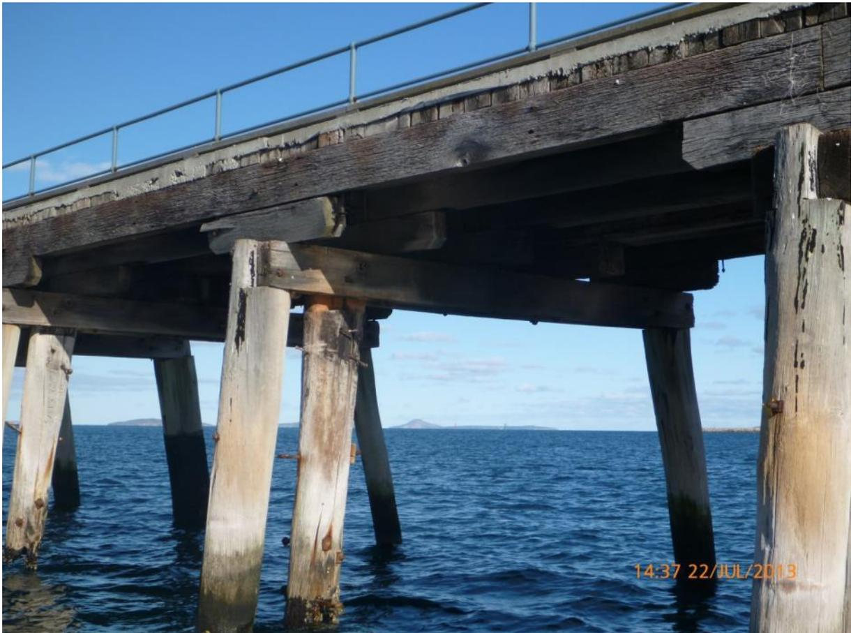
The corbel has split and rotated about the longitudinal axis. The remedial should be in order of preference where possible;
