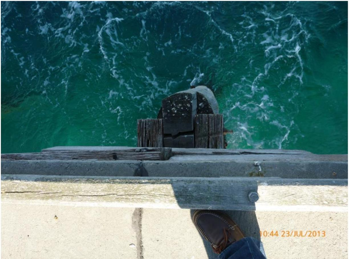
The top of the pile has split. The remedial should be in order of preference where possible;
