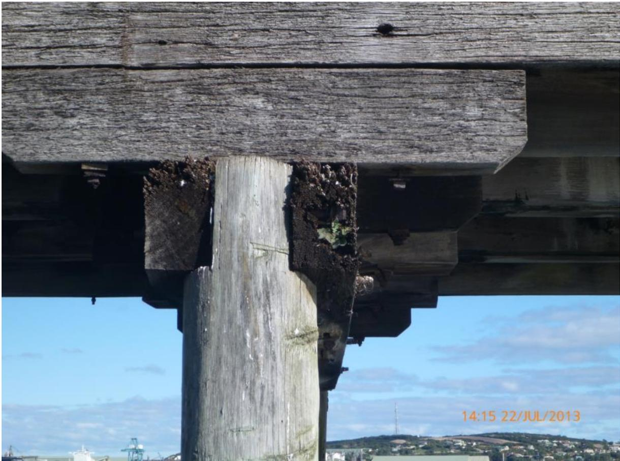
The end distance on the half cap to pile bolt connection is insufficient, and with the weathering to the half caps, the connection is no longer effective. The remedial should be;
