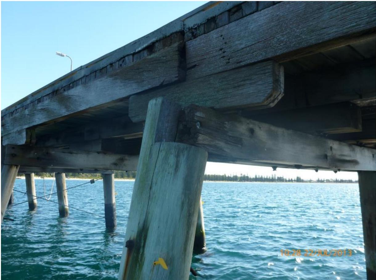
The end distance on the half cap to pile bolt connection is insufficient, and with the weathering to the half caps, the connection is no longer effective. In addition, the rot to the south-eastern half caps has reduced the bearing strength sufficiently for crushing to occur. The remedial should be in order of preference where possible;
