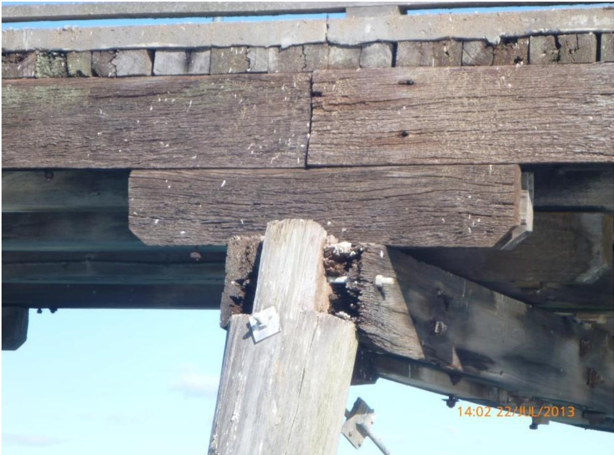
The end distance on the half cap to pile bolt connection is insufficient, and with the weathering to the half caps, the connection is no longer effective. In addition, the rot to the northern half caps has reduced the bearing strength sufficiently for crushing to occur. The remedial should be in order of preference where possible;
