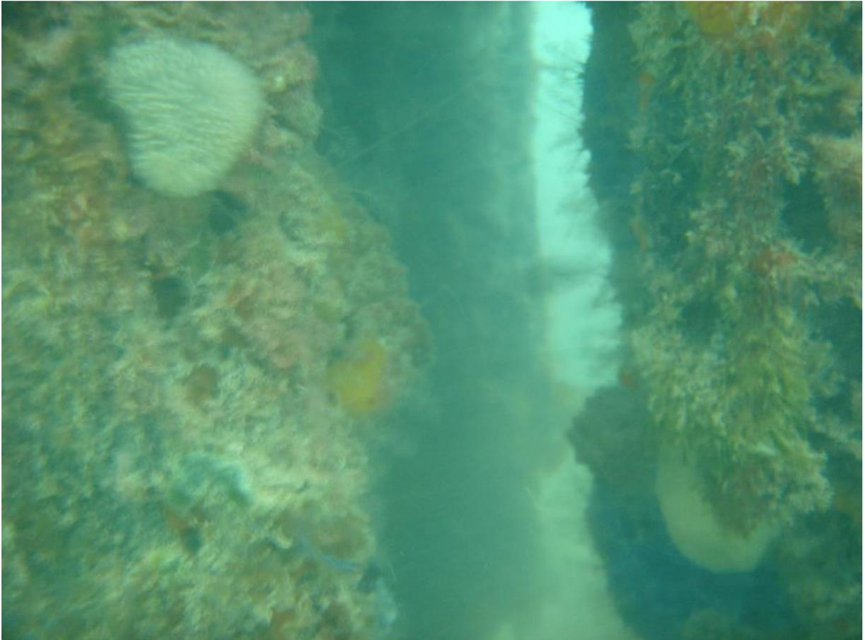
Pile 39 South has a hole through the centre of the pile (This was first encountered on the previous dive inspection – BG&E report 2010). The size of hole appears similar in size. Diver's reported that pieces of rotten timber could be broken away with fingers on one side, other side firm.
