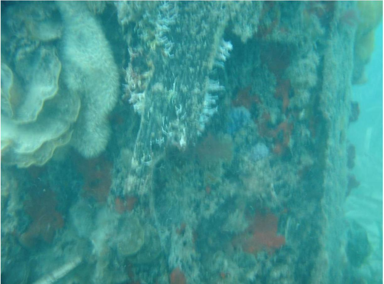
Pile 49 North has suffered some visible section loss. There is likely to be further section loss due to Teredo worm that is not visible.
