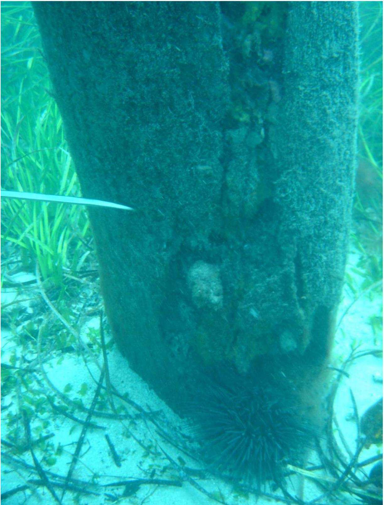
Pile 118 North has minor section loss. Divers found the affected area to be relatively solid timber with no screwdriver embedment possible.
