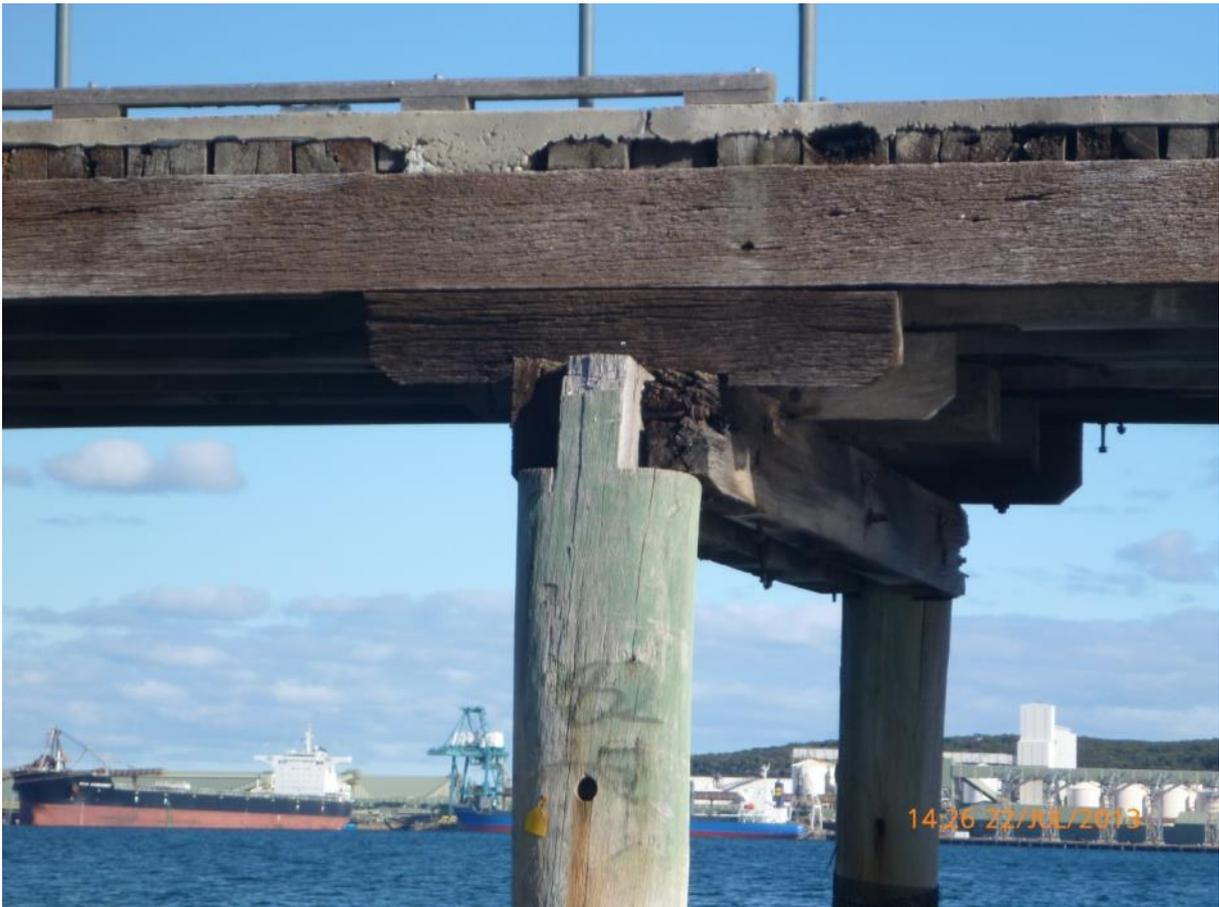
The end distance on the half cap to pile bolt connection is insufficient, and with the weathering to the half caps, the connection is no longer effective. There is evidence that the west half cap bolt has slipped in relative to the pile. The remedial should be in order of preference where possible;
