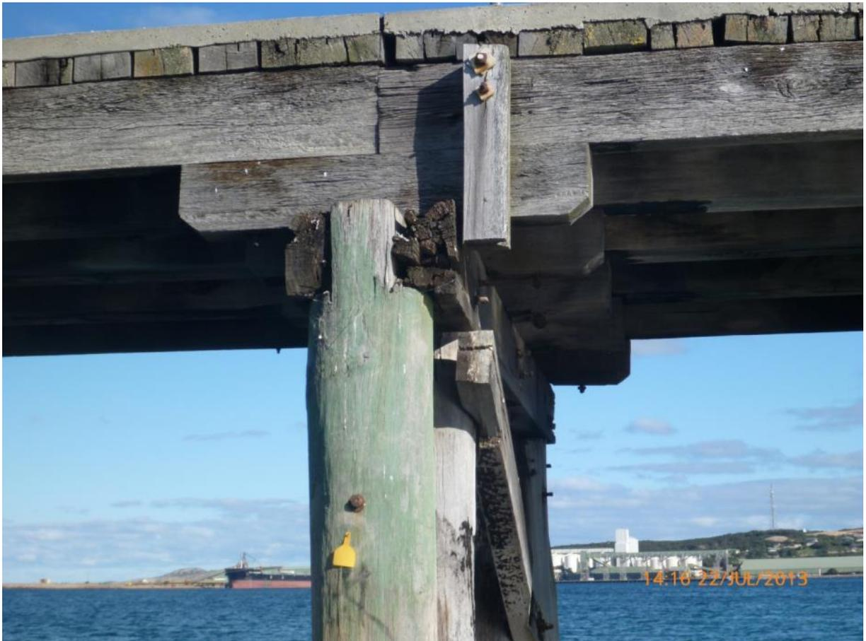
The end distance on the half cap to pile bolt connection is insufficient, and with the weathering to the half caps, the connection is no longer effective. In addition, the northwestern half cap has crushed. The north-eastern half cap appears in good condition so the bearing loads can be transferred to this element. The remedial should be in order of preference where possible;
