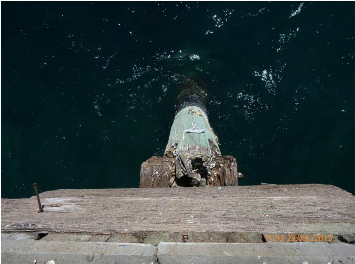
The top of the pile has lost section at the bolted interface with the half caps. The remedial should be in order of preference where possible;
