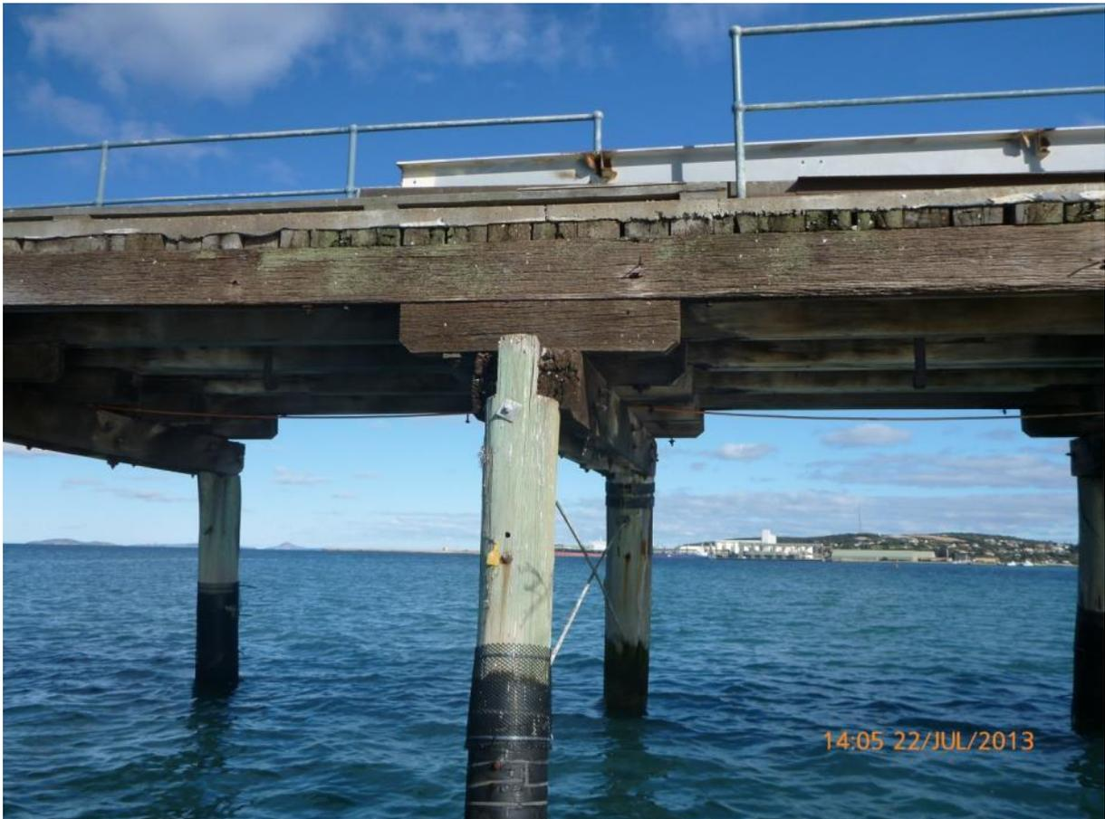
The end distance on the half cap to pile bolt connection is insufficient, and with the weathering to the half caps, the connection is no longer effective. In addition the rot to the northern half cap has reduced the bearing strength sufficiently for crushing to occur. This pier is adjacent to the missing pile which adds extra load to all elements below the bridging beam increasing the chance of failure. The remedial should be in order of preference where possible;
