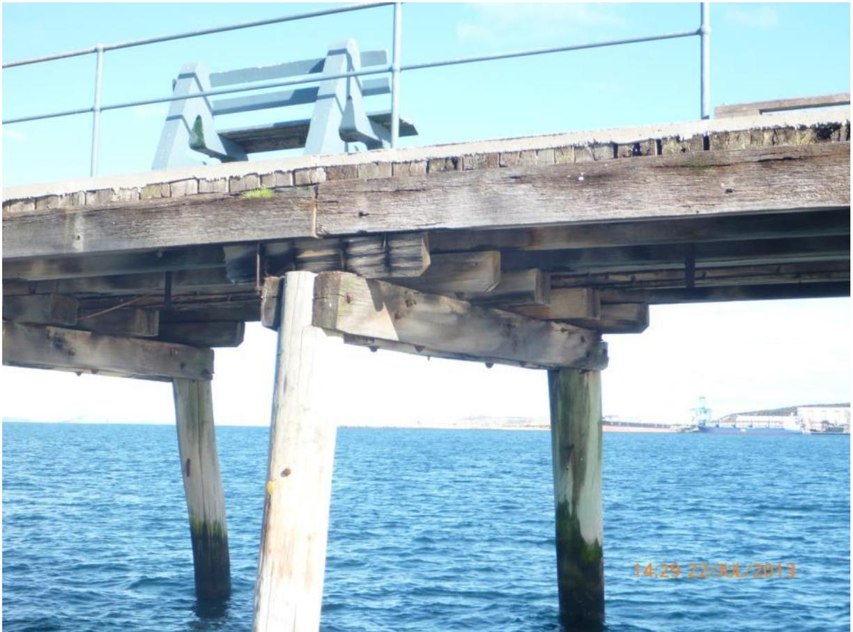
The corbel has split with loss of half of section. The remedial should be in order of preference where possible;
