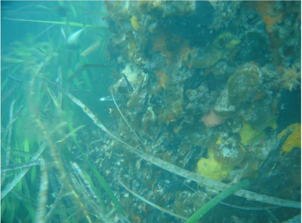
Pile 49 South has suffered some visible section loss. There is likely to be further section loss due to Teredo worm that is not visible.
