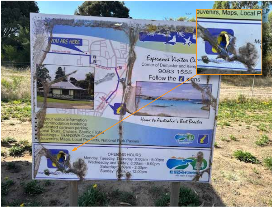
South Coast Hwy - Poorly produced ancillary sign promoting the Esperance Visitor Centre, vinyl has failed and there is a large hole in the bottom left-hand corner
