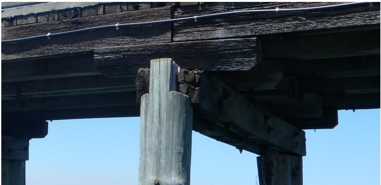
Figure 3-19: 43 North 17/11/15 – Crushing of both half caps
