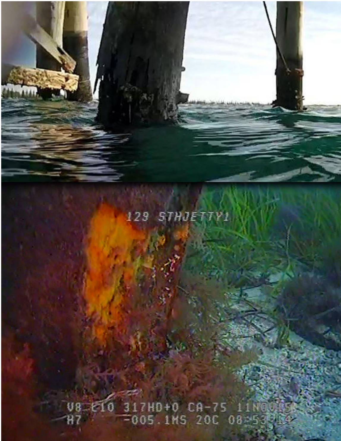
Figure 3-12: 129 South 11/11/15 – Severe section loss at surface (top), section loss at base (bottom)
