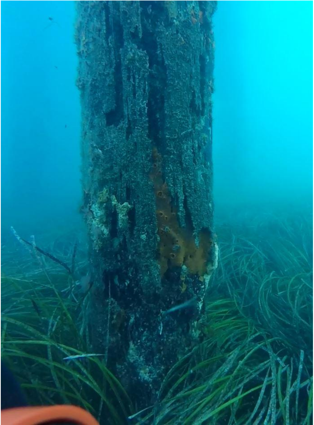
Figure 3-11: 112 North 11/11/15 – Severe section loss at base
