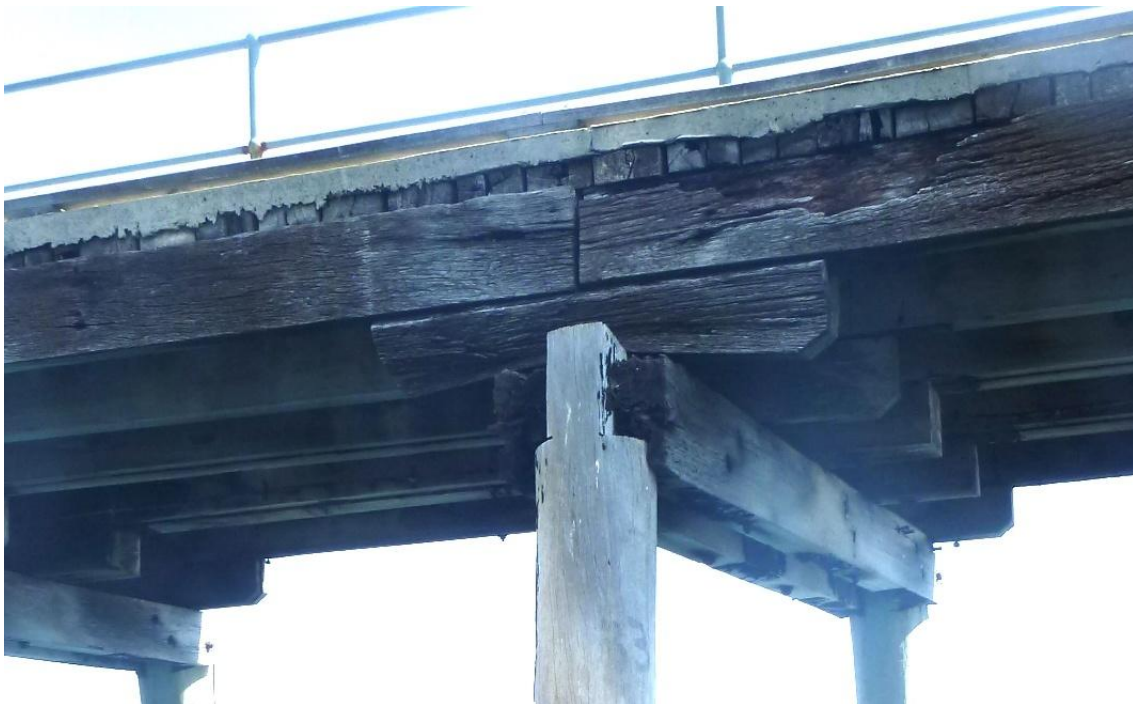
Figure 3-23: 133 North 17/11/15 – Crushing of both half caps
