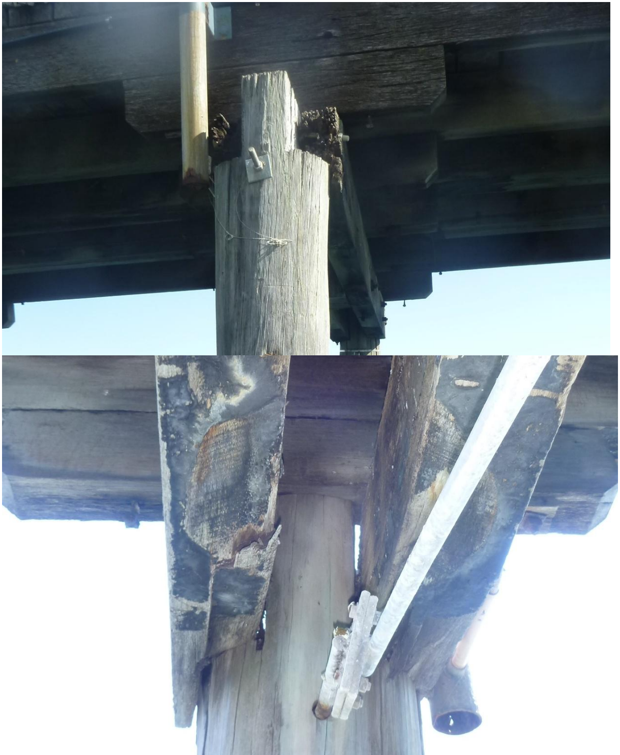
Figure 3-15: 36 North 17/11/15 – Crushing of both half caps
