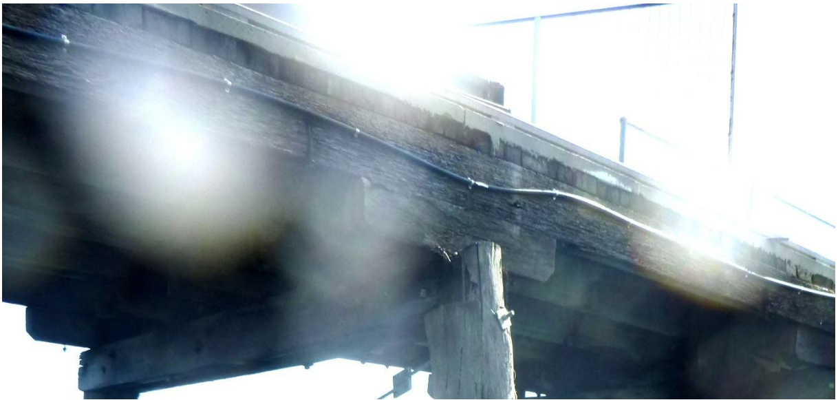
Figure 3-17: 38 North 17/11/15 – Crushing of both half caps
