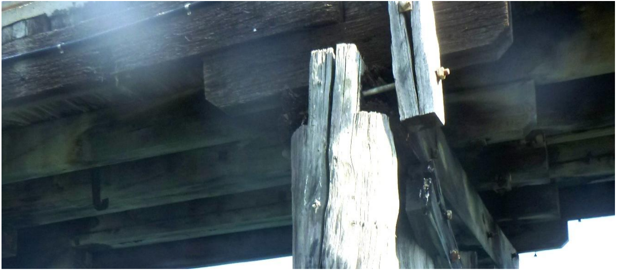
Figure 3-16: 37 North 17/11/15 – Crushing of both half caps
