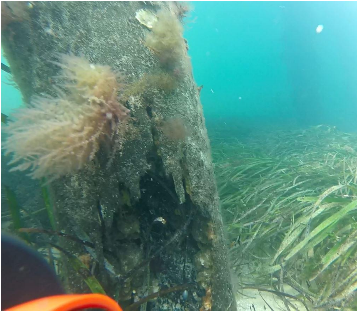
Figure 3-4: 58 South 11/11/15 – Severe section loss at base
