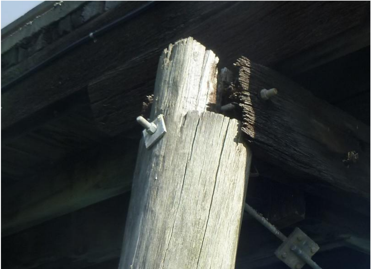
Figure 3-14: 35 North West 17/11/15 – Crushing of both half caps
