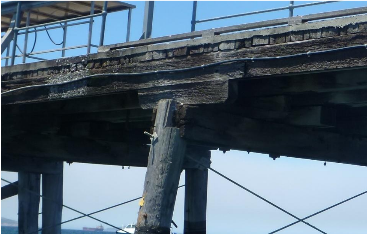
Figure 3-20: 43 North 17/11/15 – Crushing of both half caps
