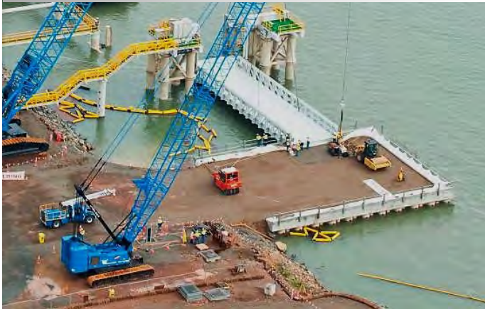
GLNG – RG Tanna - RoRo Facility during construction Superlift Manitowoc crane installing the linkspan bridge (110t) as a single crane lift
