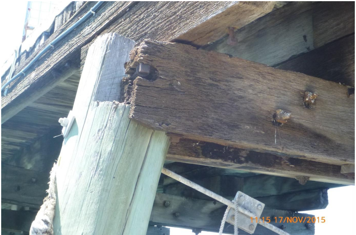
Figure 3-18: 40 North 17/11/15 – Crushing of both half caps
