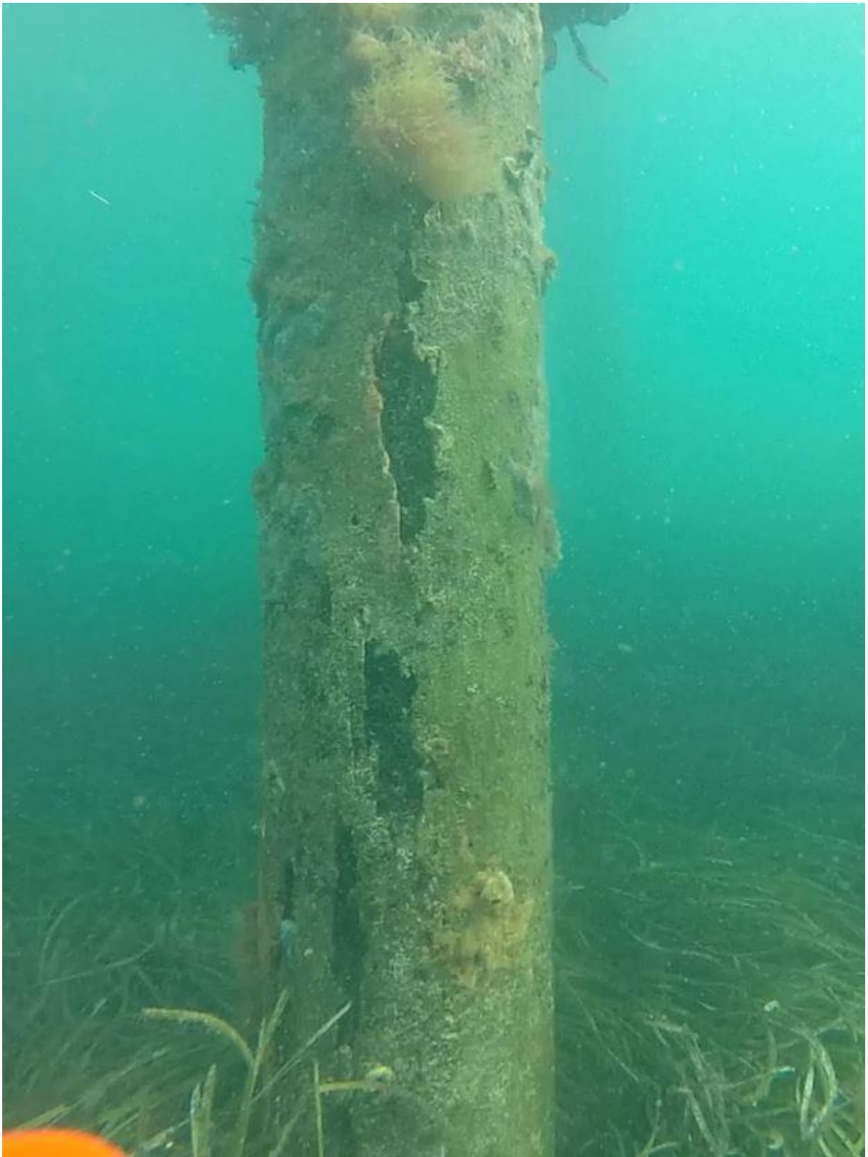
Figure 3-8: 74 North 11/11/15 – Section loss and splitting at many locations through water column
