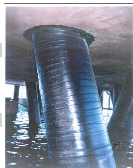
▲ Figure 1. Denso Seashield Series 60 system (excluding Pilemesh).
