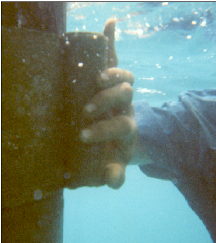
▲ Figure 3. Tape being applied under water.
