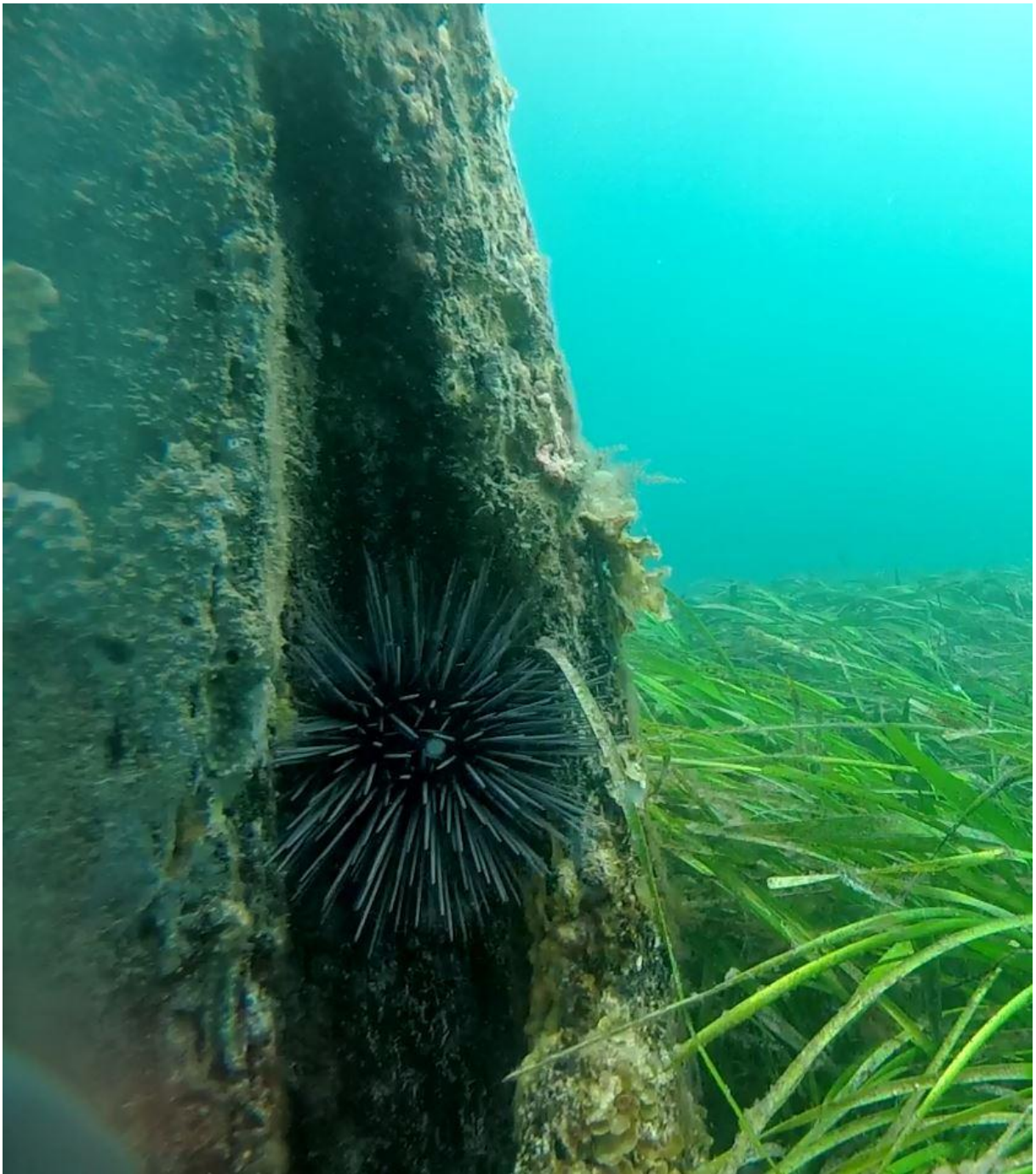
Figure 3-10: 101 North 11/11/15 – Severe section loss at base
