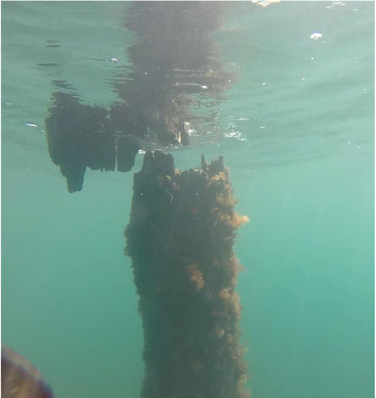
Figure 3-2: 93 North 11/11/15 – Failure at surface
