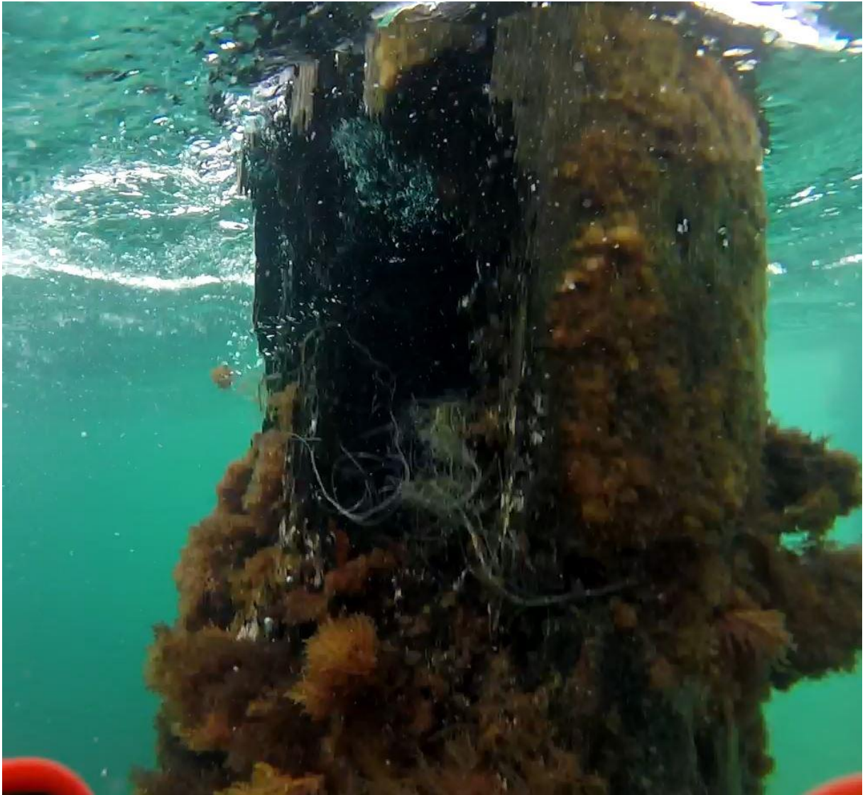
Figure 3-3: 53 South 11/11/15 – Severe section loss at surface
