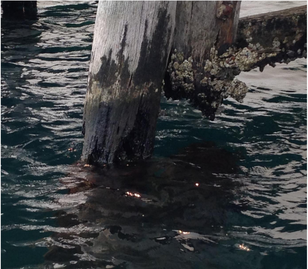
Figure 3-6: 70 South 17/11/15 – Severe section loss at surface (surface inspected only)
