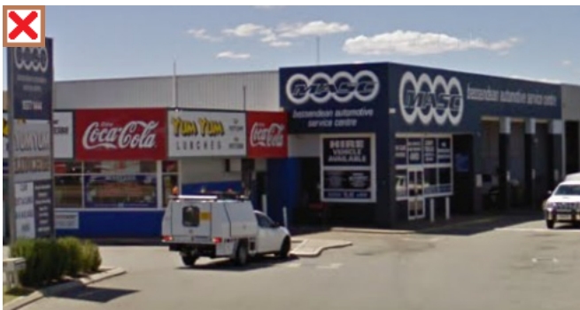
Messy advertising signs detract from the amenity of the area.
