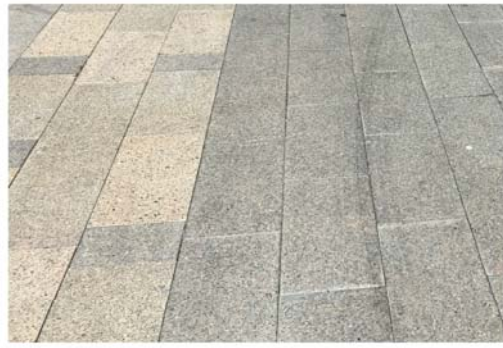
EXISTING GRANITE PAVER IN FORESHORE AREA (SUITABLE FOR POSTOFFICE SQUARE AND OTHER SPECIAL URBAN AREAS)
