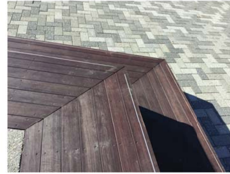
TIMBER SEATING DECK (POST OFFICE SQUARE AND (SUITABLE FOR OTHER SPECIAL URBAN AREAS))
