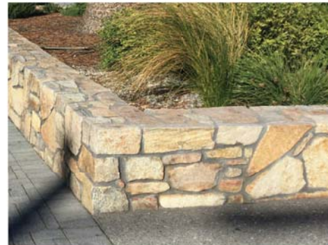
GRANITE STONE WALL (LOCAL GRANITE) ( ROUNDABOUT ANDREW STREET / DEMPSTER STREET)
