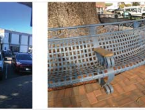
BENCH & PAVING AROUND THE BASE OF NORFOLK ISLAND TREE CONTRIBUTE TO COMPACTION AND LACK OF NUTRITION SUPPLY (POST OFFICE SQUARE)
