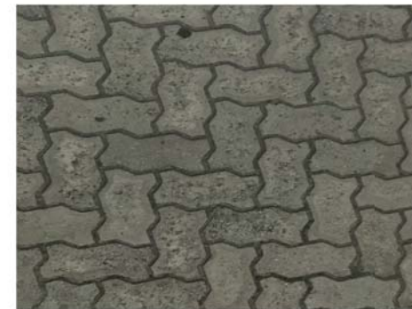
EXISTING CONCRETE PAVER IN CBD (PEDESTRIAN PATHWAY)
