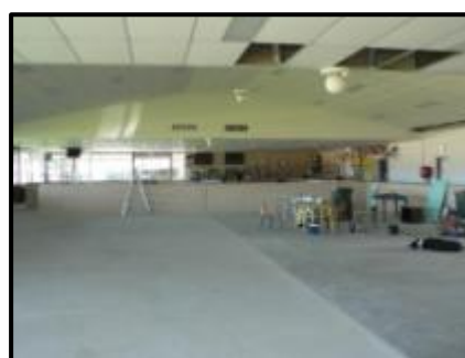
Social Facilities being upgraded
