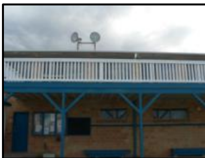
Front view of building
