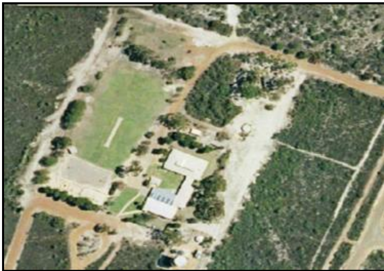
Condungup Primary School Aerial View
