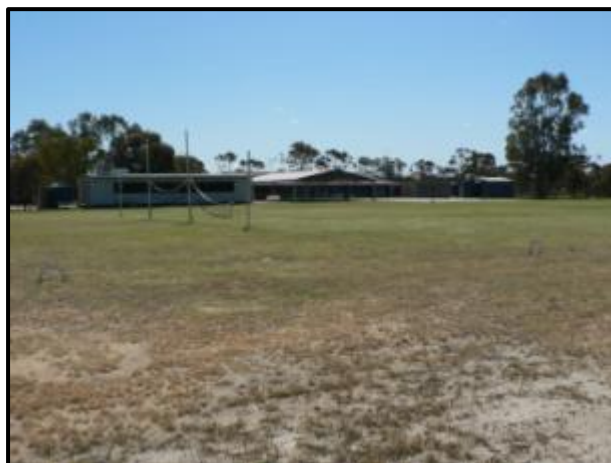
Oval and Part Covered Hard Court
