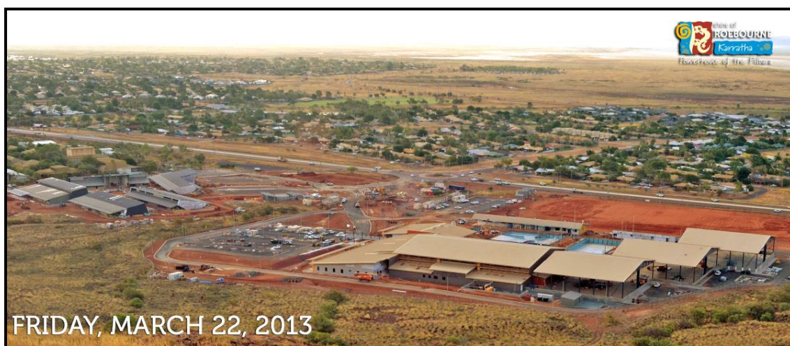
Karratha Leisureplex under construction
