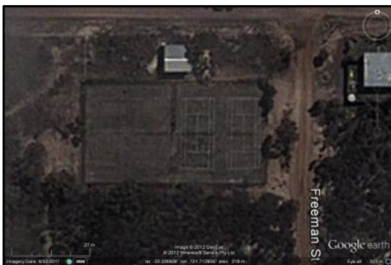
Aerial View of Tennis Courts (pre-refurbishment)
